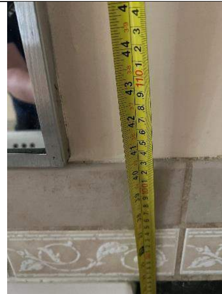
PHOTO #44: Mirror height of 41 inches in men's restroom on second floor (Compliant).
