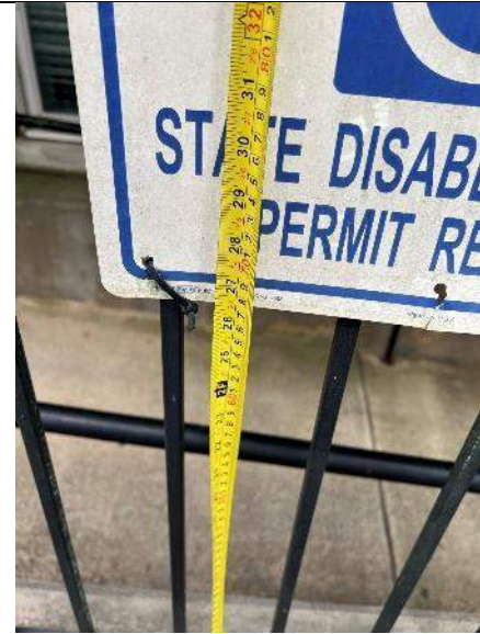
PHOTO #14: Signage height is 27" (Non-Compliant). Signs are required to be mounted a minimum of 60" above the grade of the parking space.
