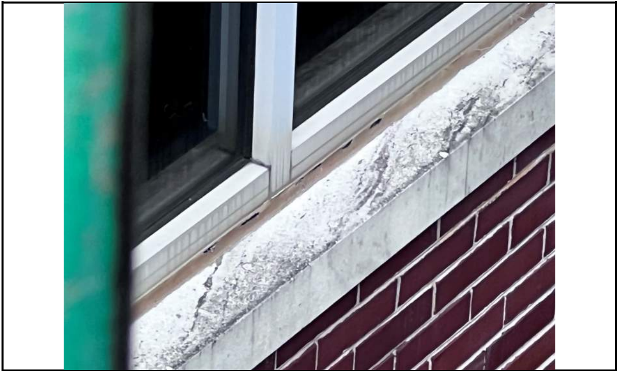
Photo 51: Adhesive failure of sealant around aluminum framed window systems
