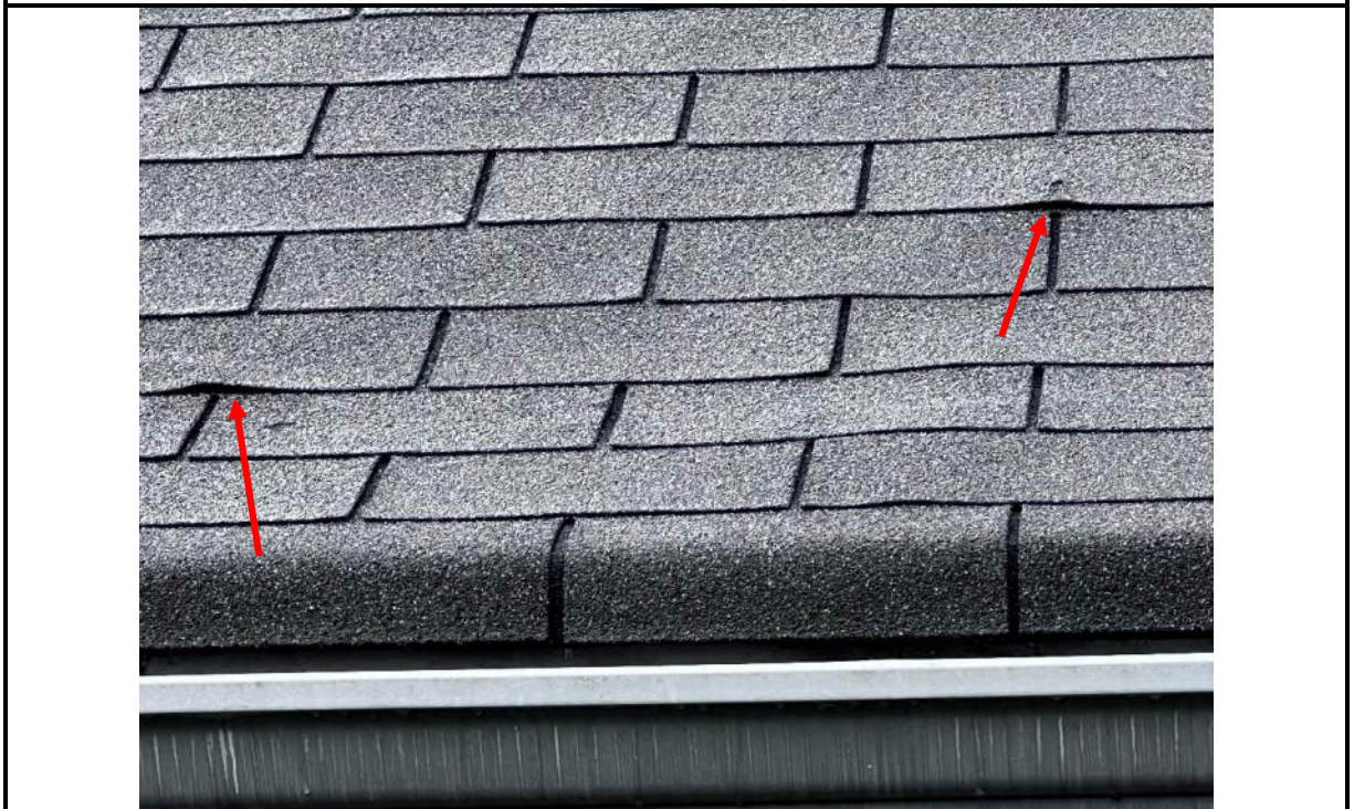
Photo 72: Shingle nails beginning to backout and raise the shingle tab above.
