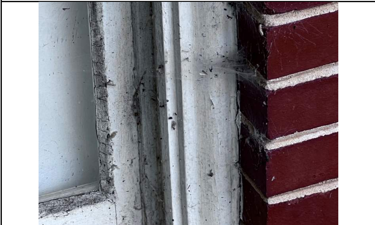
Photo 46: Cracked glazing putty, typical most wood window frames
