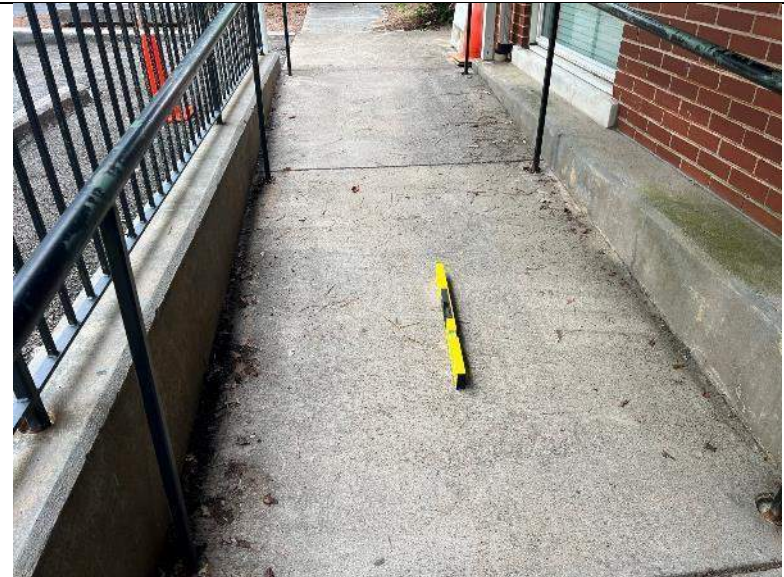
PHOTO #12: Edge protection is provided along full ramp run.
