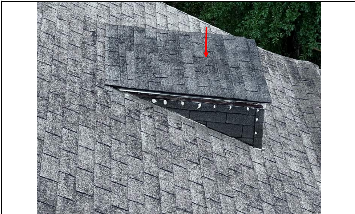
Photo 73: Roof pop-up dormer, insufficient slope for shingles
