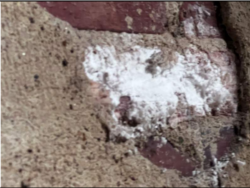
Photo 3: Efflorescence on interior side of exterior backed masonry wall.
