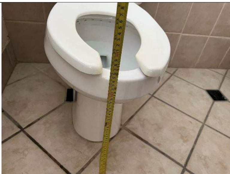
PHOTO #47: Toilet height of 18" in men's restroom on second floor (Compliant).
