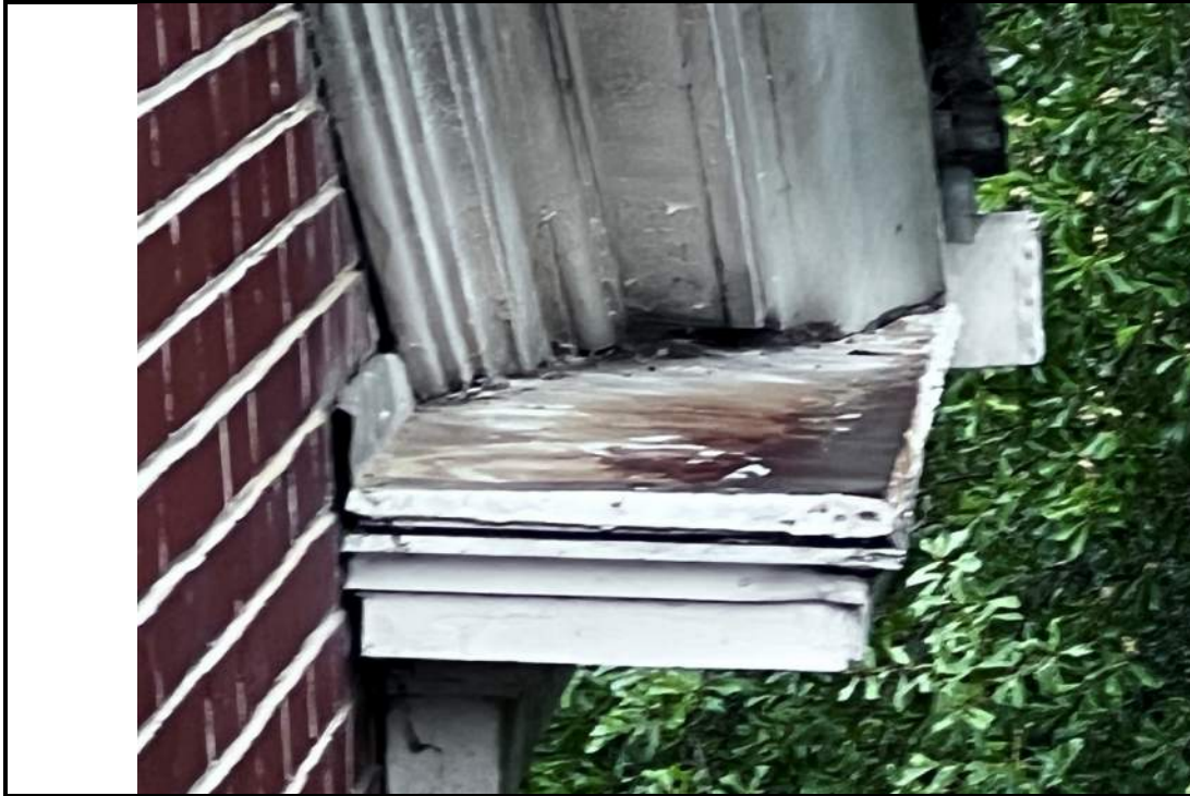
Photo 65: Metal cornice return cap exhibits some corrosion
