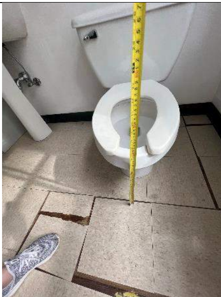
PHOTO #55: Toilet height of 16" (Non-Compliant).
