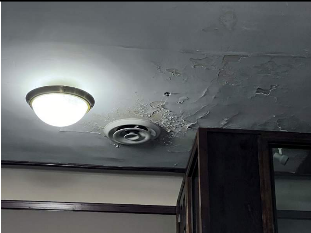
Photo 14: Apparent water damage above balcony.
