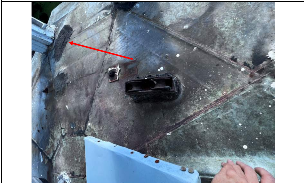
Photo 58: Previous repairs performed are temporary in nature and need to be maintained
