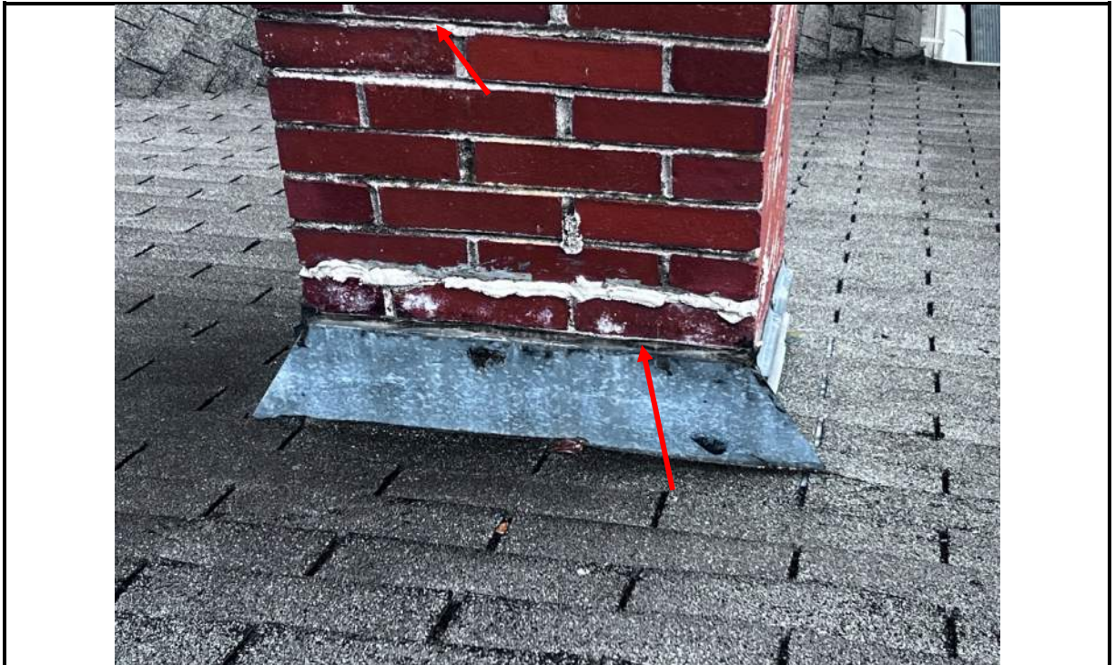
Photo 77: Chimney counter flashing exhibited deteriorated sealant as well as mortar erosion
