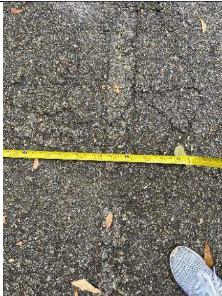
PHOTO #15: Access aisle width measurement of 82" (Compliant).
