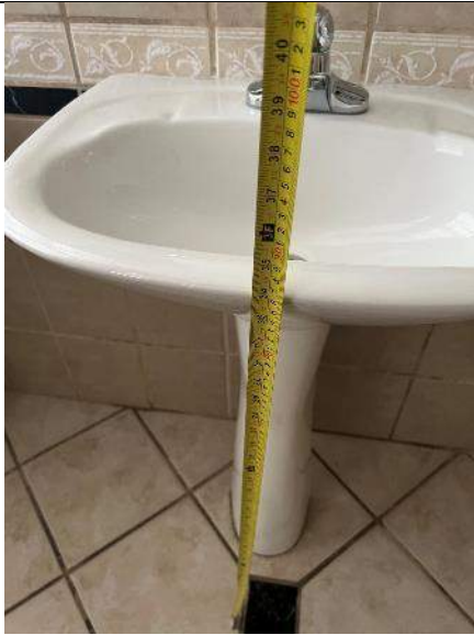
PHOTO #37: Sink height of 34" in women's restroom second floor. (Compliant)
