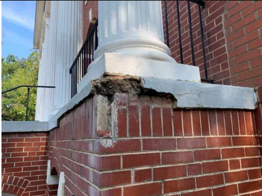
Photo 4: Observed missing elevated concrete slab material and brick facade near south main entrance columns.
