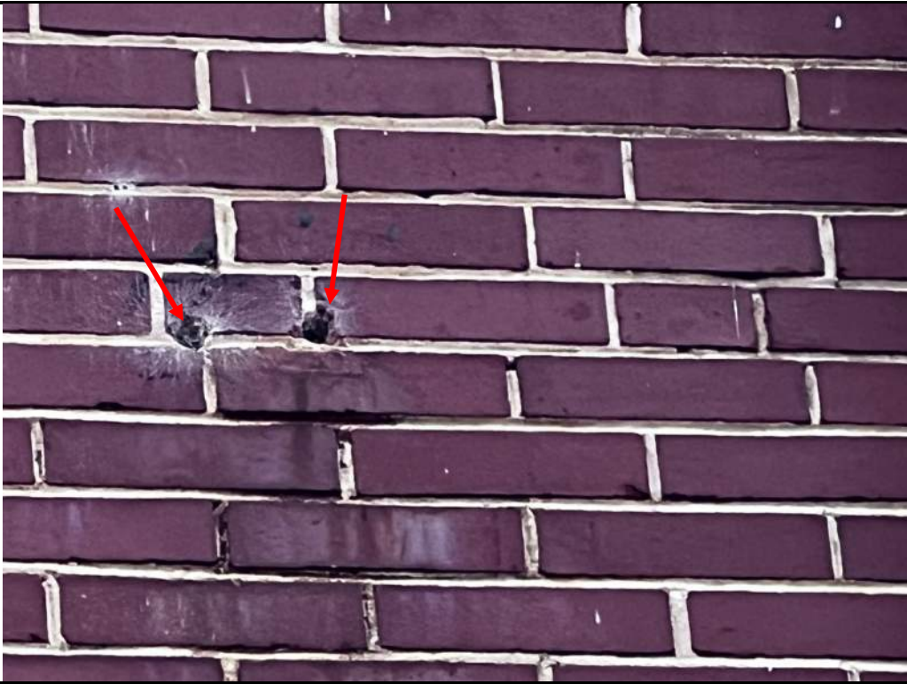
Photo 33: Spalled masonry brick because of performing penetrations.
