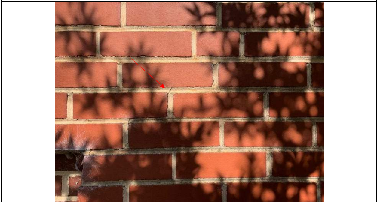
Photo 8: Isolated, low-severity stair-step crack in exterior brick façade.
