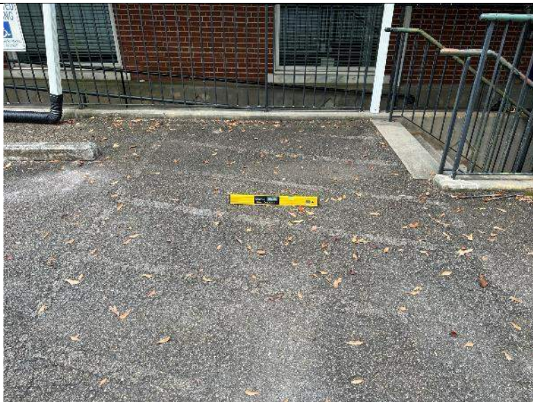
PHOTO #19: Cross slope of access aisle being obtained.
