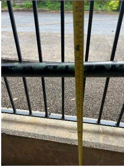
PHOTO #9: Height of gripping surface at railing on ramp is 35". (Compliant).
