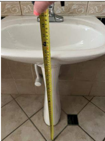
PHOTO #45: Sink height of 34" in men's restroom on second floor (Compliant).
