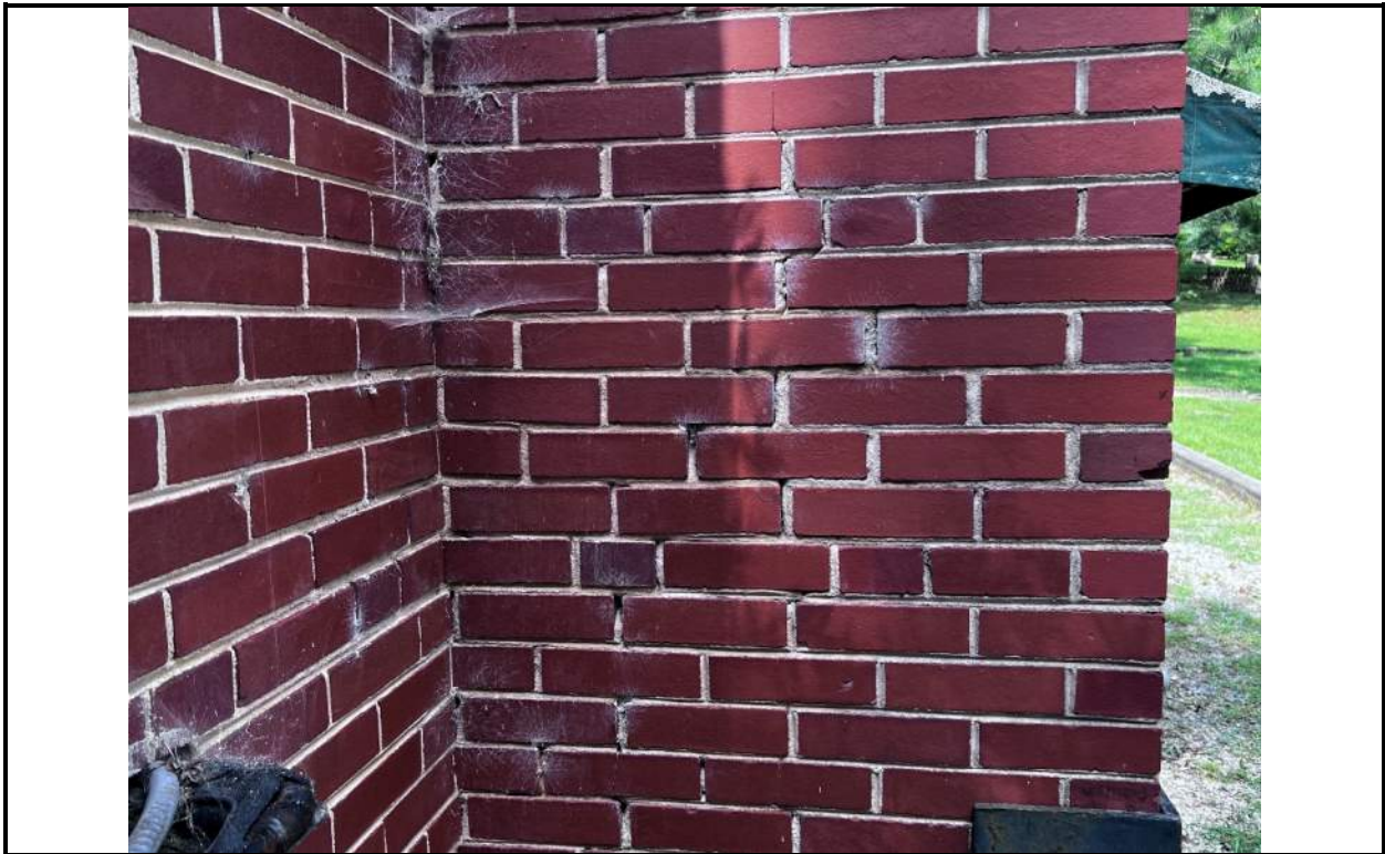
Photo 35: Deteriorating mortar
