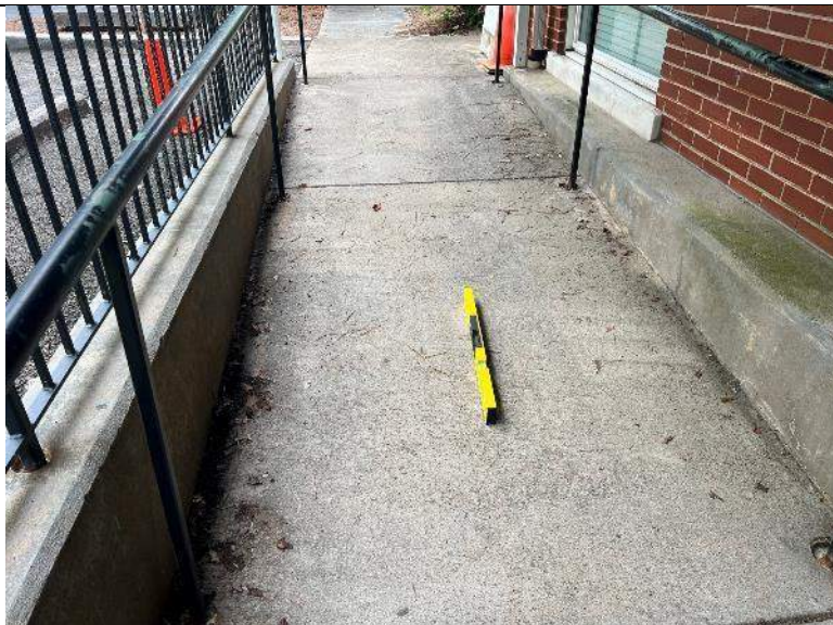
PHOTO #5: View running slope being obtained along ramp.
