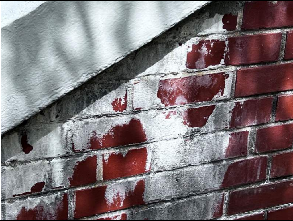
Photo 27: Efflorescence and lime staining on face of brick
