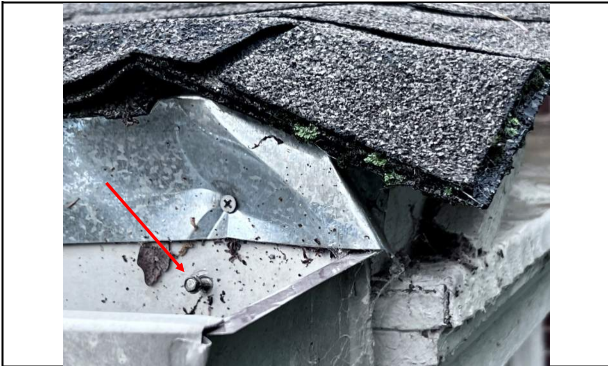
Photo 63: Poorly performed edge metal flashing, also note loose gutter screw
