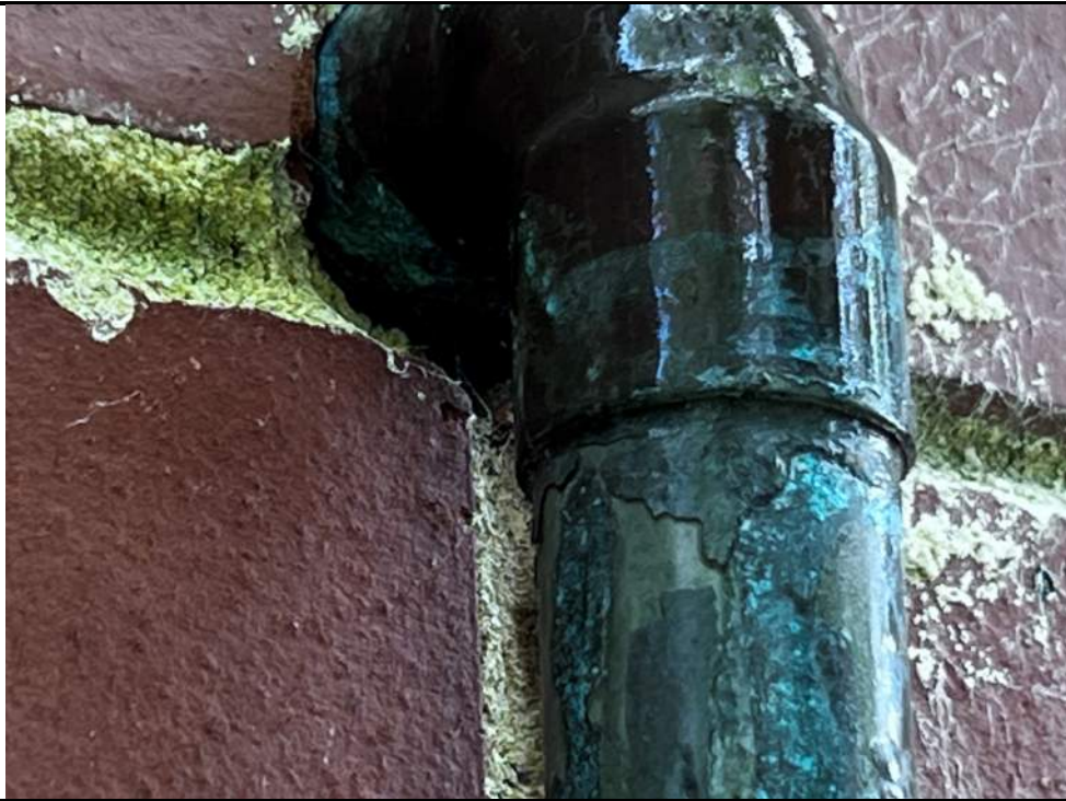
Photo 41: Unsealed wall penetration
