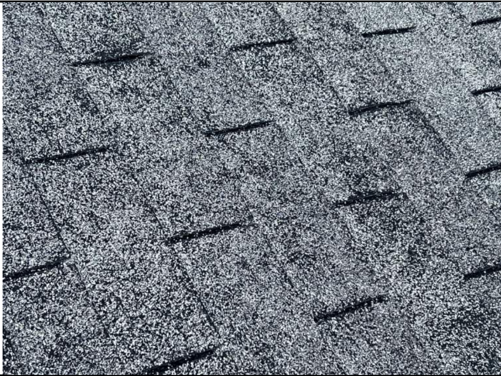
Photo 69: Erosion of ceramic granules from shingle surface
