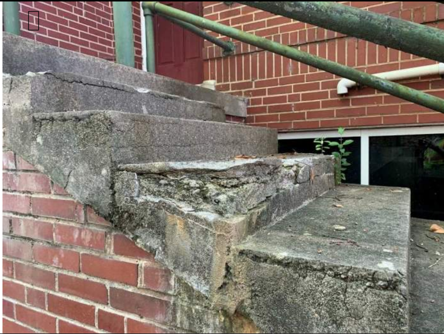
Photo 11: Observed severely damaged concrete stairs. Significant repair or remove and replace required.
