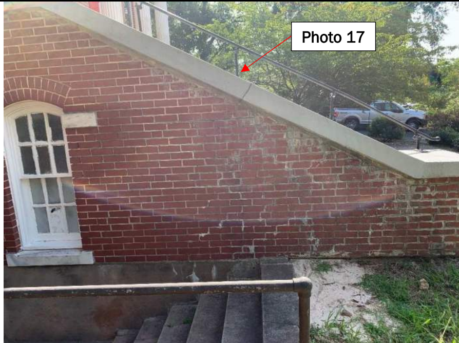
Photo 15: Overview of south entrance stairwell to ground floor. Recommend tuckpoint repair of exterior brick.
