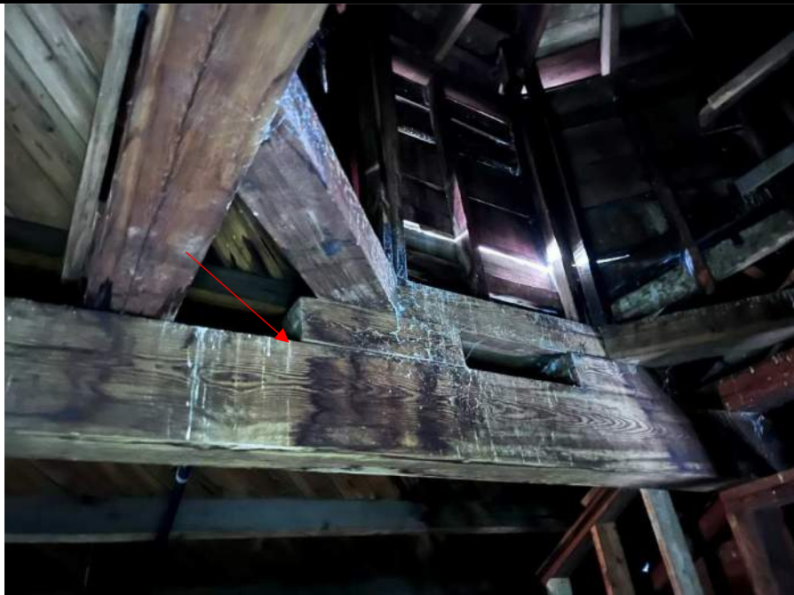
Photo 30: Observed signs of previous water infiltration near the steeple near the south end of the structure.
