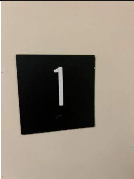
PHOTO #29: Tactile star not provided at floor signage. (Non-Compliant).
