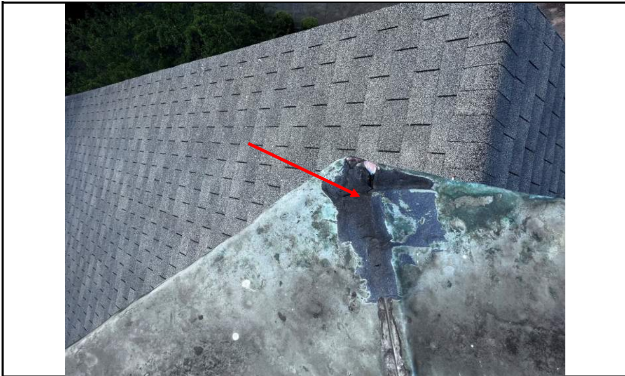
Photo 59: Previous repairs performed are temporary in nature and need to be maintained
