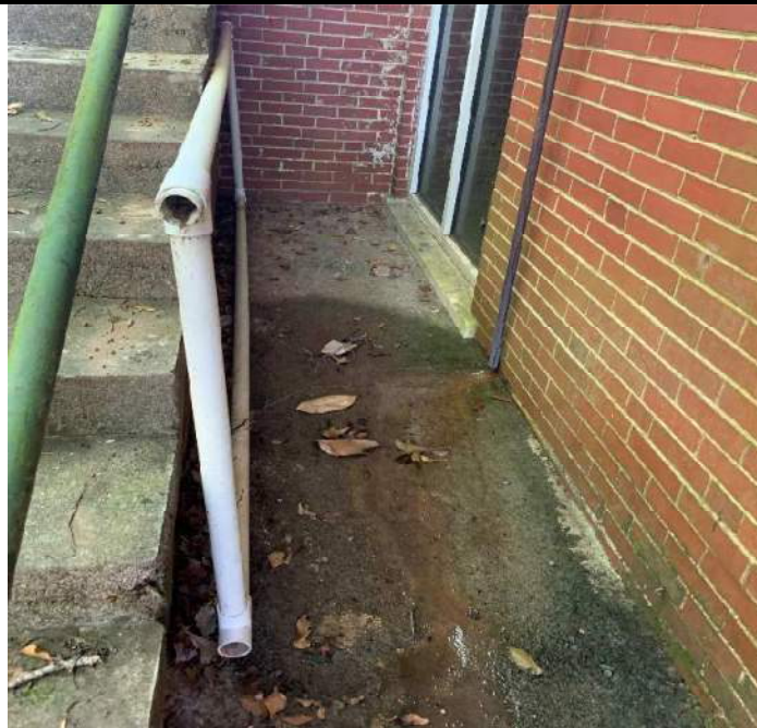
Photo 12: Subject structure concrete drain adjacent to concrete stairs, observed ponding of water runoff from roof drain system.
