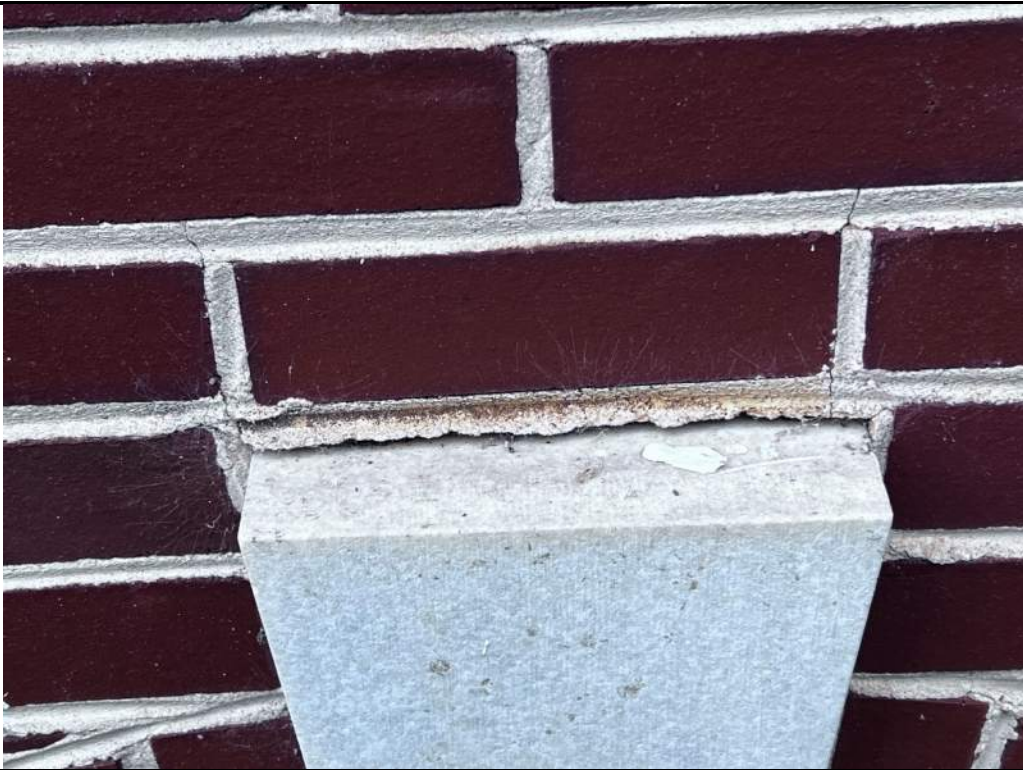
Photo 29: Keystone believed to be loose above aluminum framed arched window
