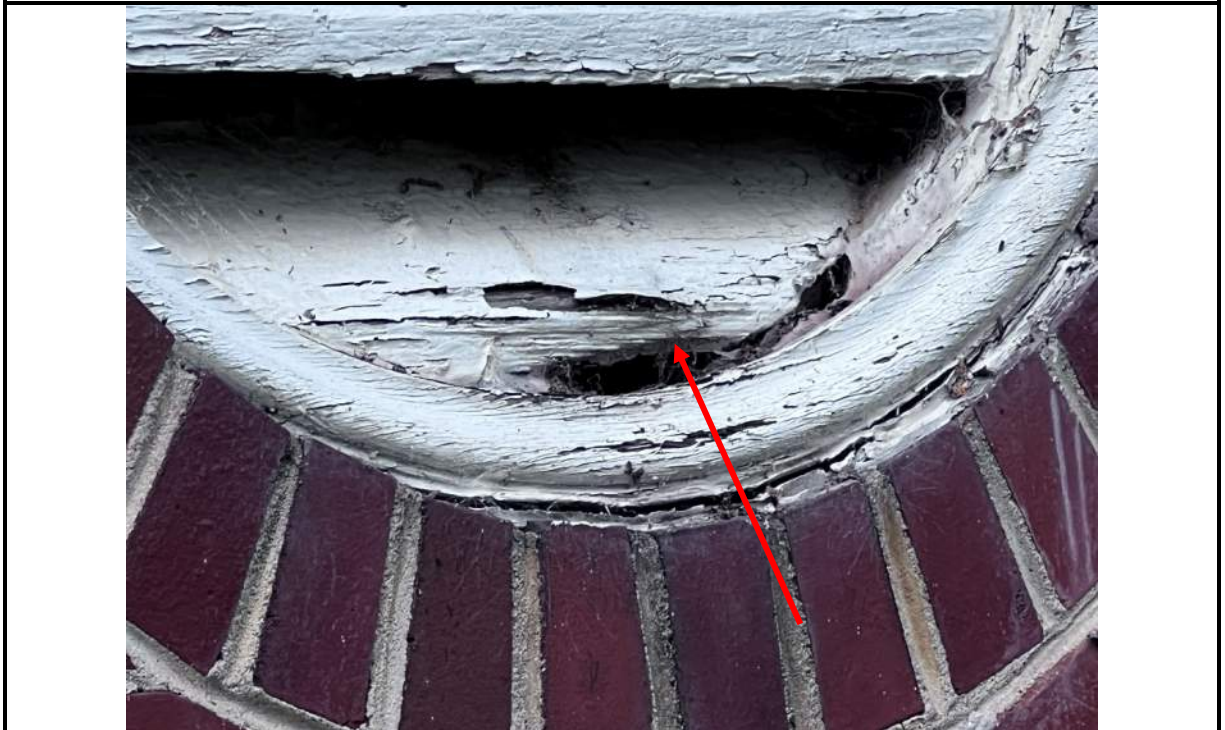
Photo 50: Deteriorated wood gable vent, perimeter sealant is also in a deteriorated condition
