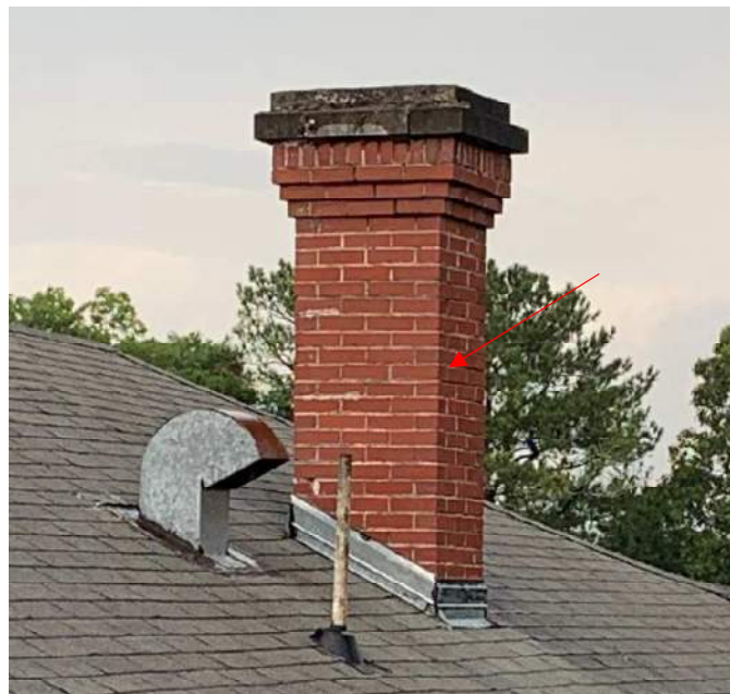
Photo 28: Overview of brick chimney near north portion of shingle roof. Observed spalls and separation in joints. Recommend tuckpoint repair.
