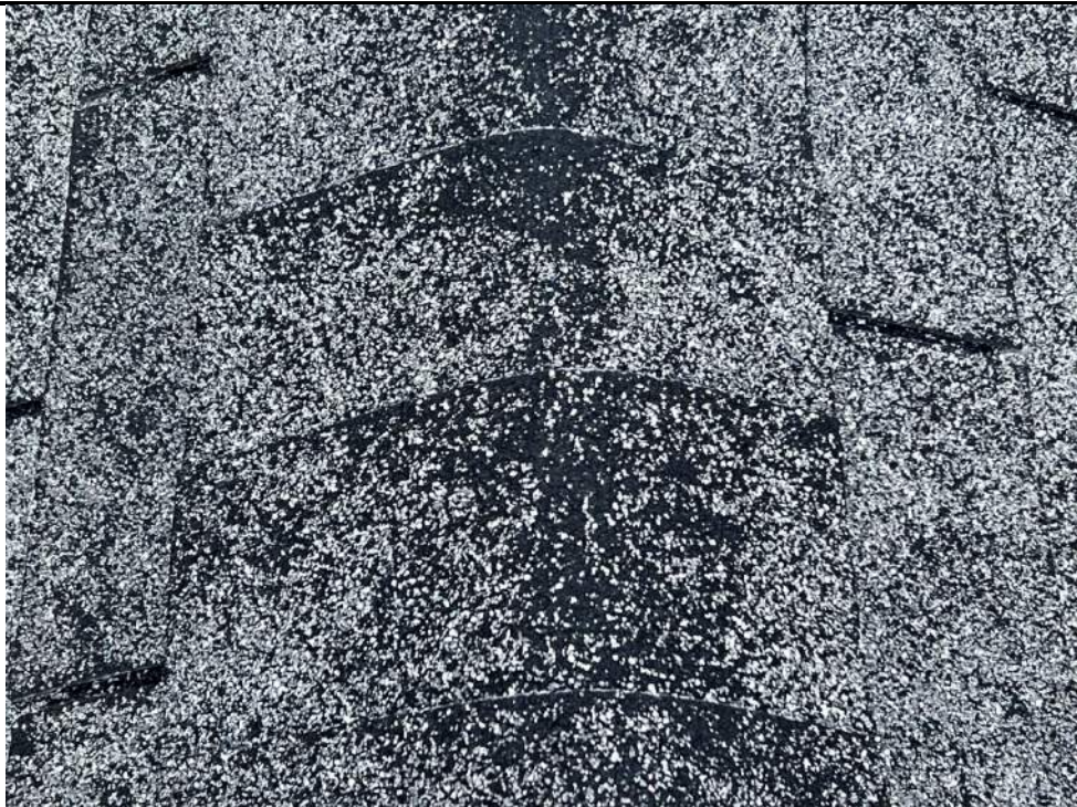
Photo 67: Erosion of ceramic granules from shingle surface
