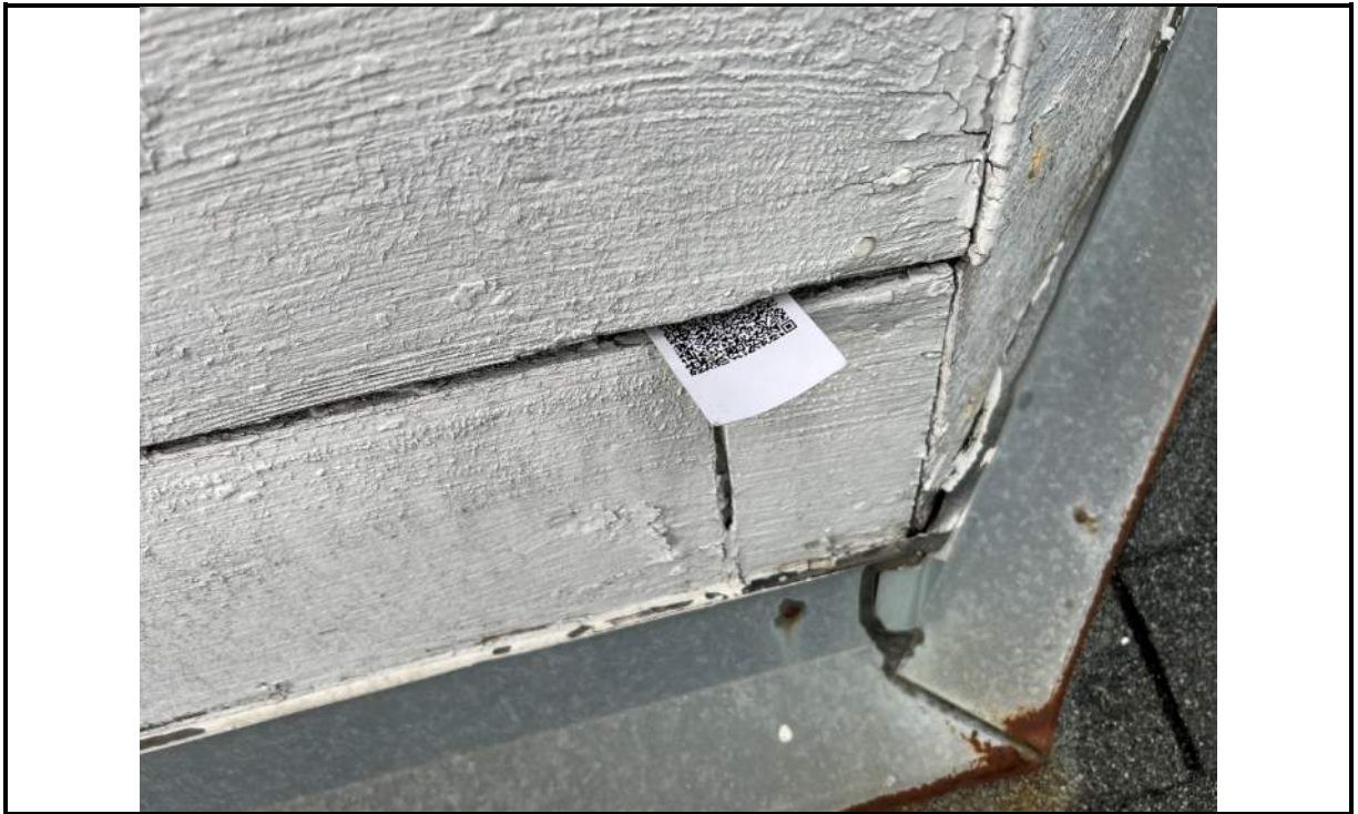
Photo 61: Steeple exterior wall panel in location of visible light in attic space (ref. photo 15)
