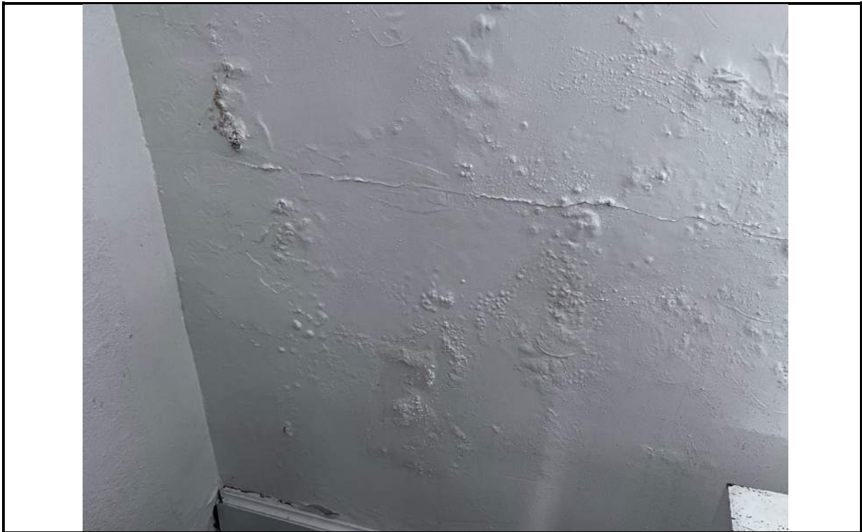
Photo 5: Blistered paint filled with efflorescence.
