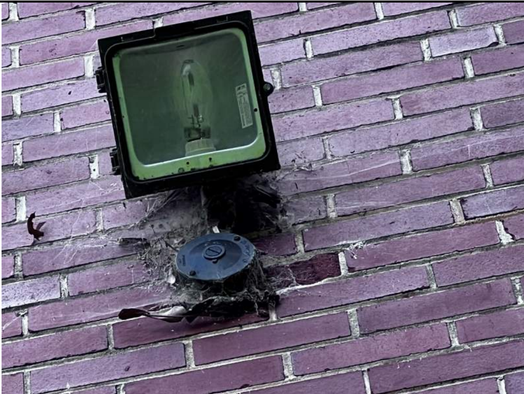
Photo 34: Spalled brick, possibly occurring during fixture installation.
