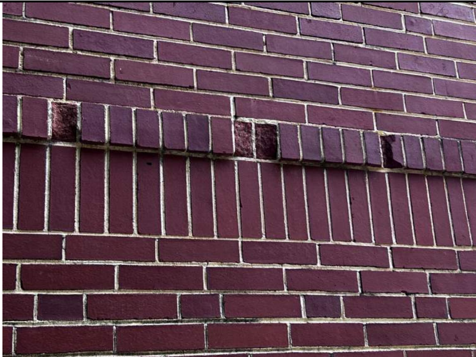
Photo 42: Spalled brick Rowlock band
