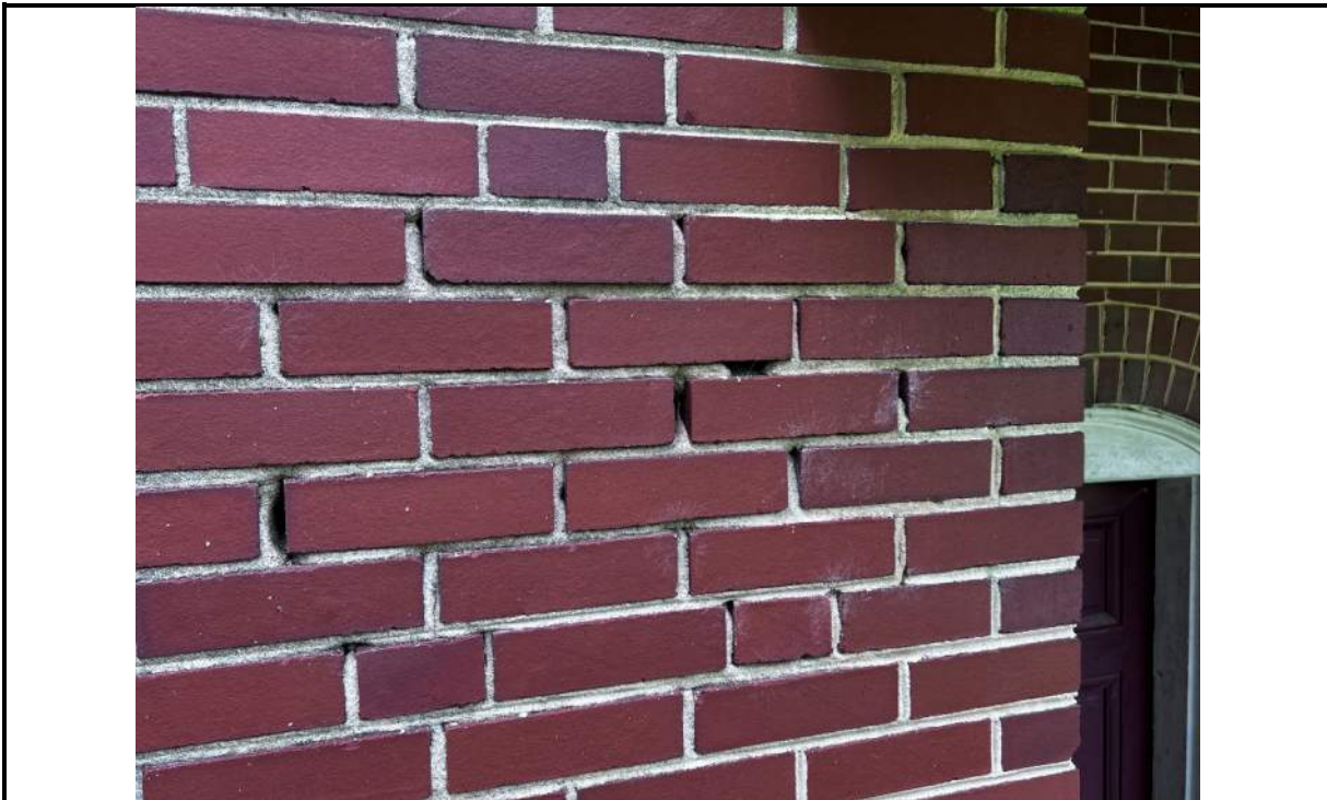
Photo 37: Eroded and missing mortar, in vicinity of wall damage in basement level mechanical room
