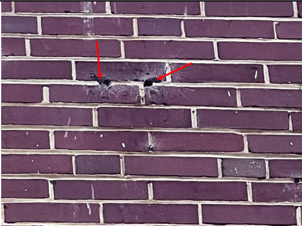
Photo 32: Spalled masonry brick because of performing penetrations
