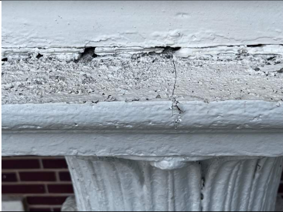
Photo 87: Small crack in the top of the column capital.
