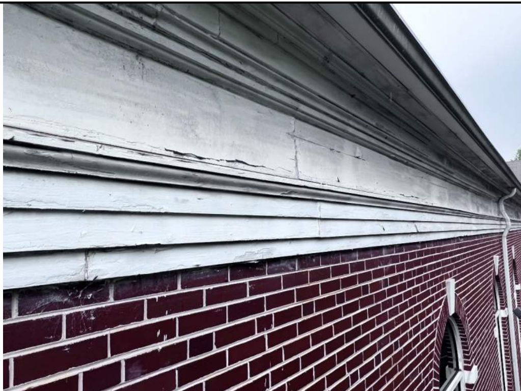
Photo 30: Paint peeling from wood fascia
