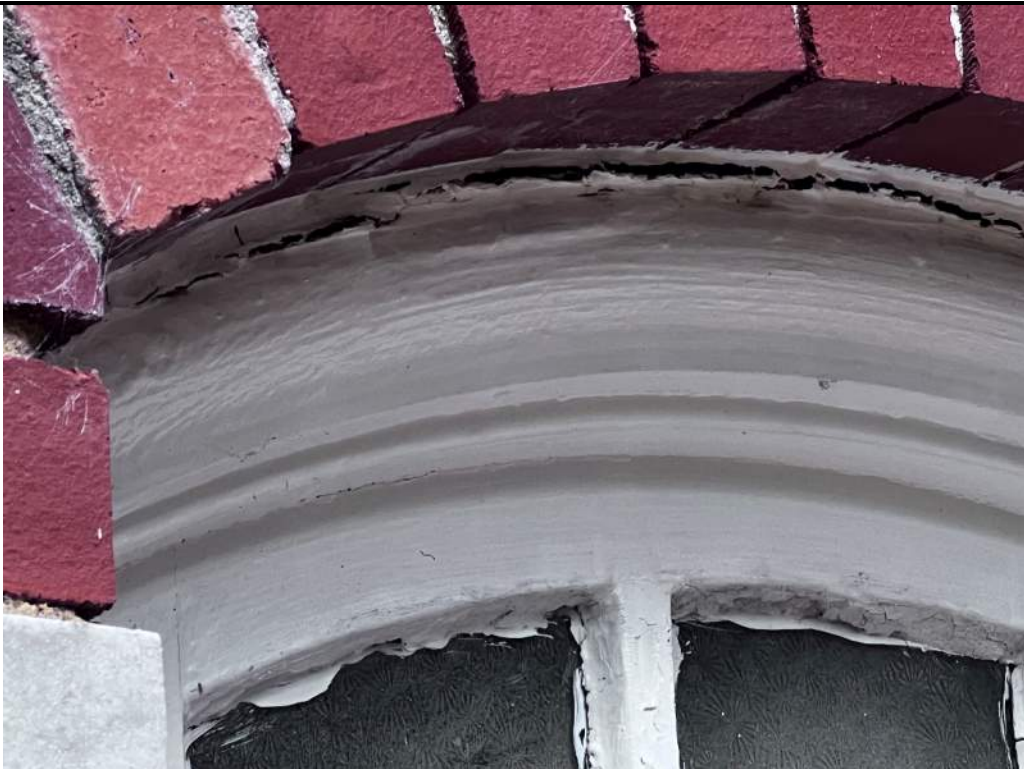
Photo 24: Perimeter sealant around window, poor condition
