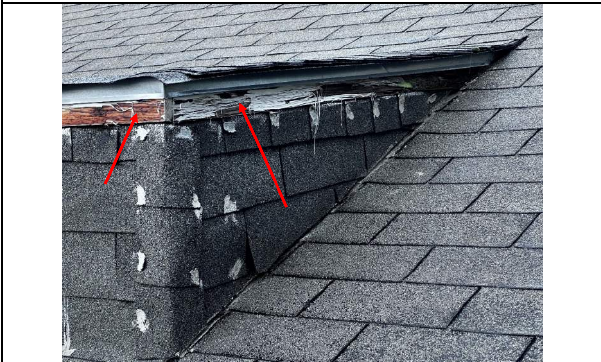
Photo 74: Exposed and deteriorated wood on 3-sides of popped up area
