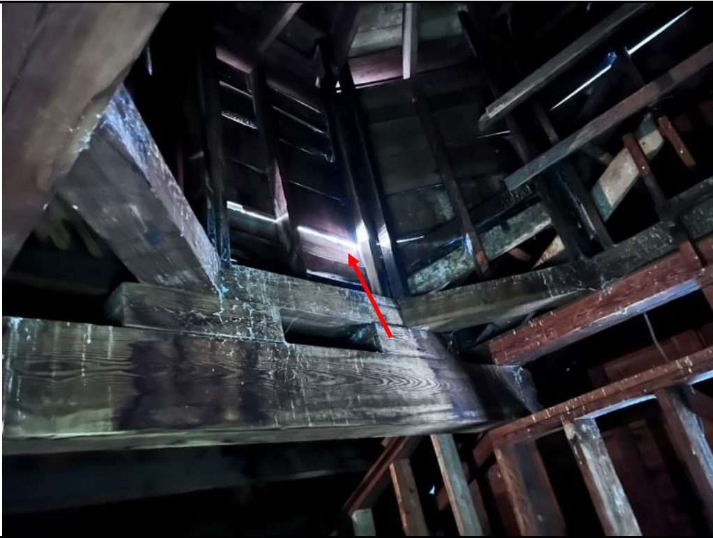
Photo 15: Open lap in steeple wood siding in close proximity to balcony leaks
