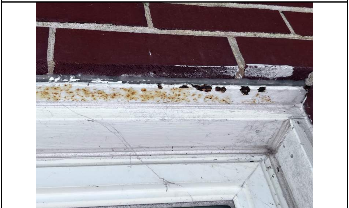
Photo 52: Many lintels above windows exhibit some metal corrosion
