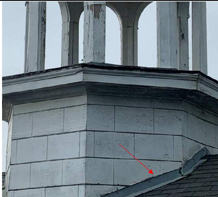
Photo 27: Overview of steeple near south elevation. Flashing appears to be in fair condition with slight corrosion. Recommend prime, and paint wood components. Remove and replace of rotten wood near flashing material as required.
