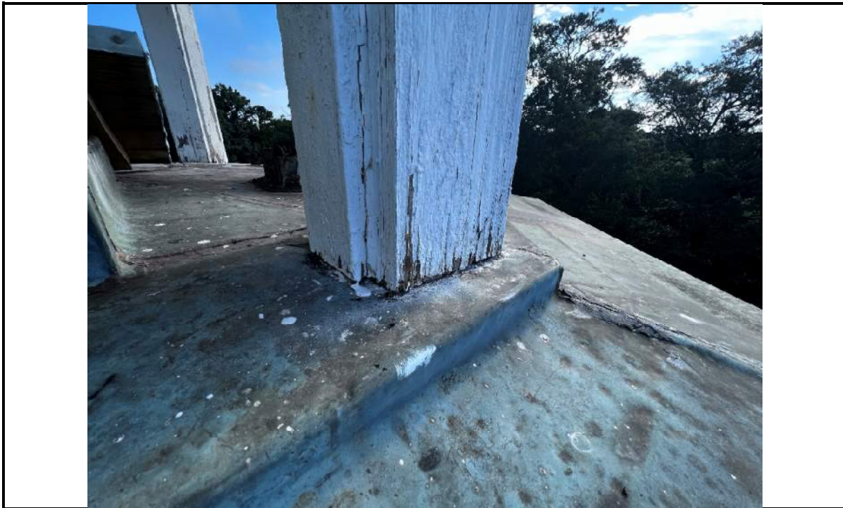
Photo 57: Steel roof support post exhibiting weathering and cracking
