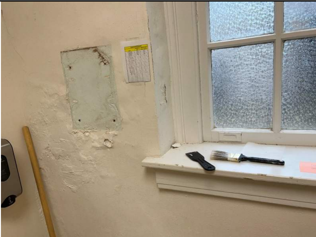
Photo 12: Blistered paint, efflorescence, men's restroom south side.
