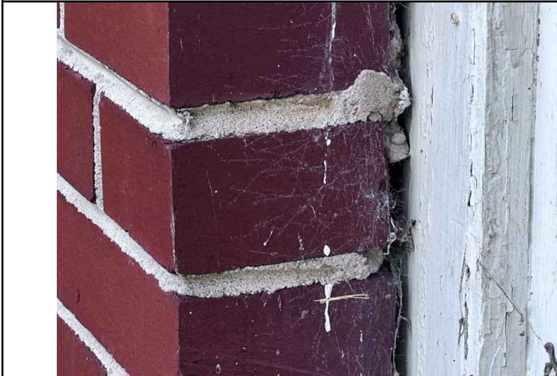
Photo 26: Open joint between masonry and wood window frame.
