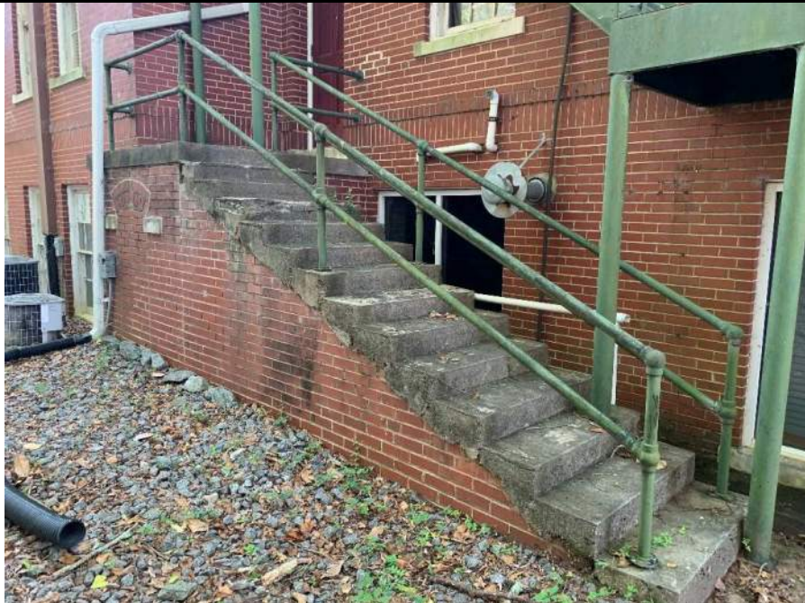
Photo 9: Overview of northwest corner exterior stairs emanating from first floor to grade. Note, handrail does not meet current building code requirements.
