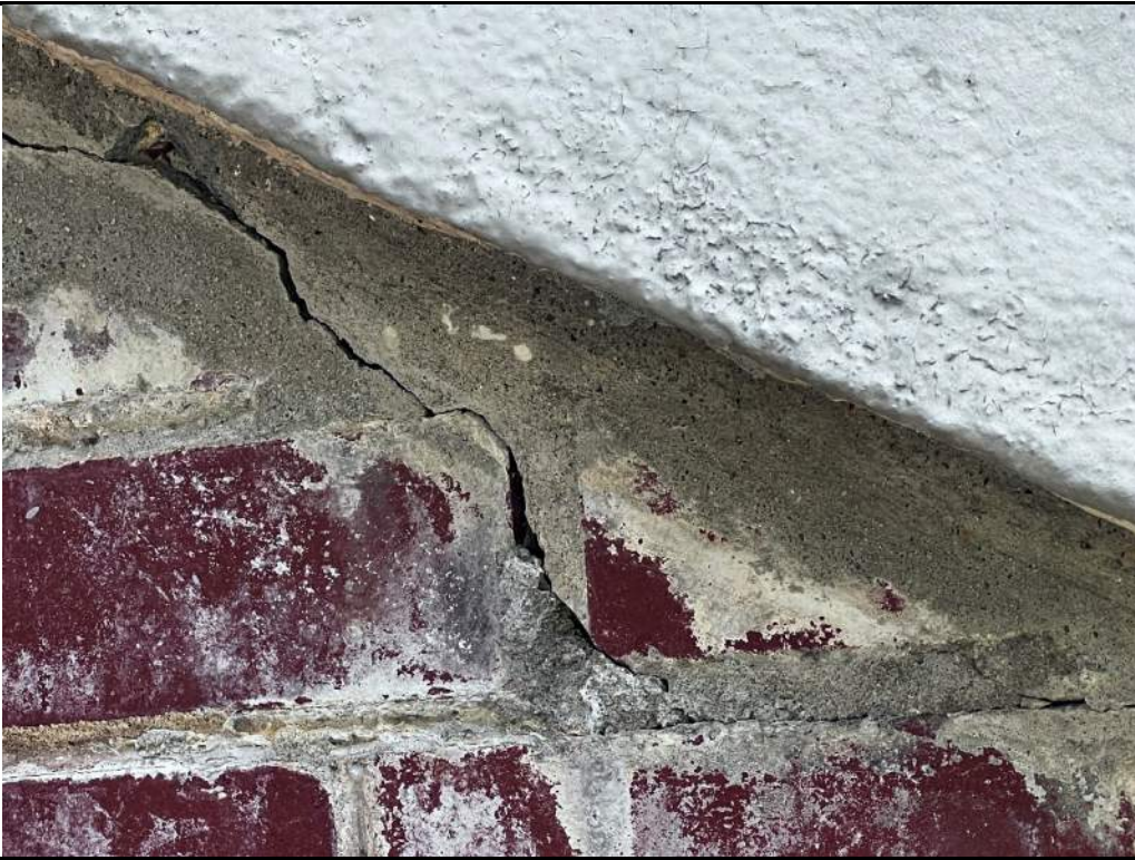
Photo 21: Cracked bed joint below concrete coping
