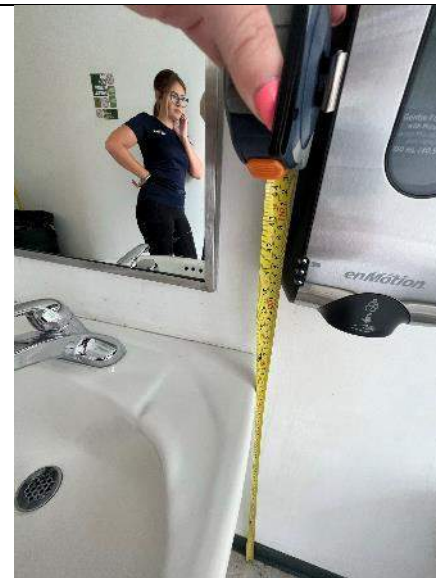
PHOTO #56: Mirror and soap dispenser height at 40" (Compliant).
