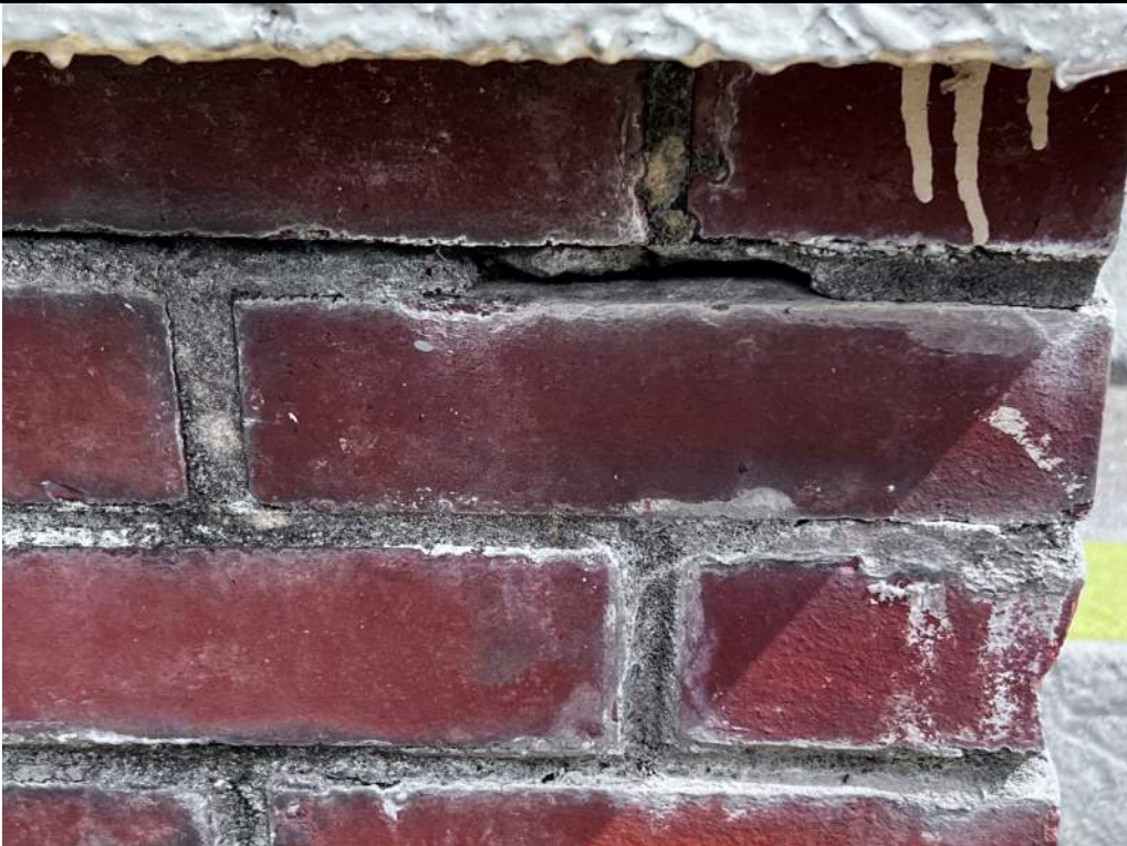
Photo 22: Brick mortar joint below concrete coping open
