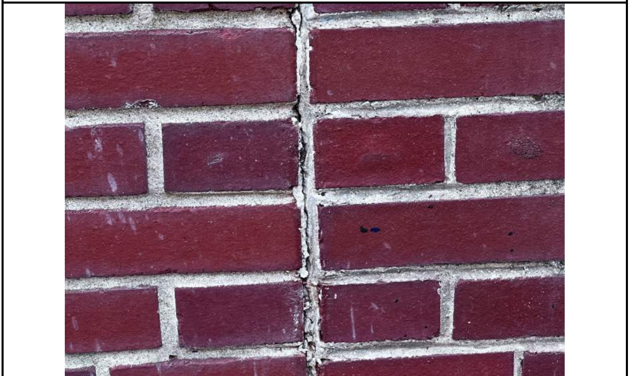
Photo 40: Deteriorated control joint
