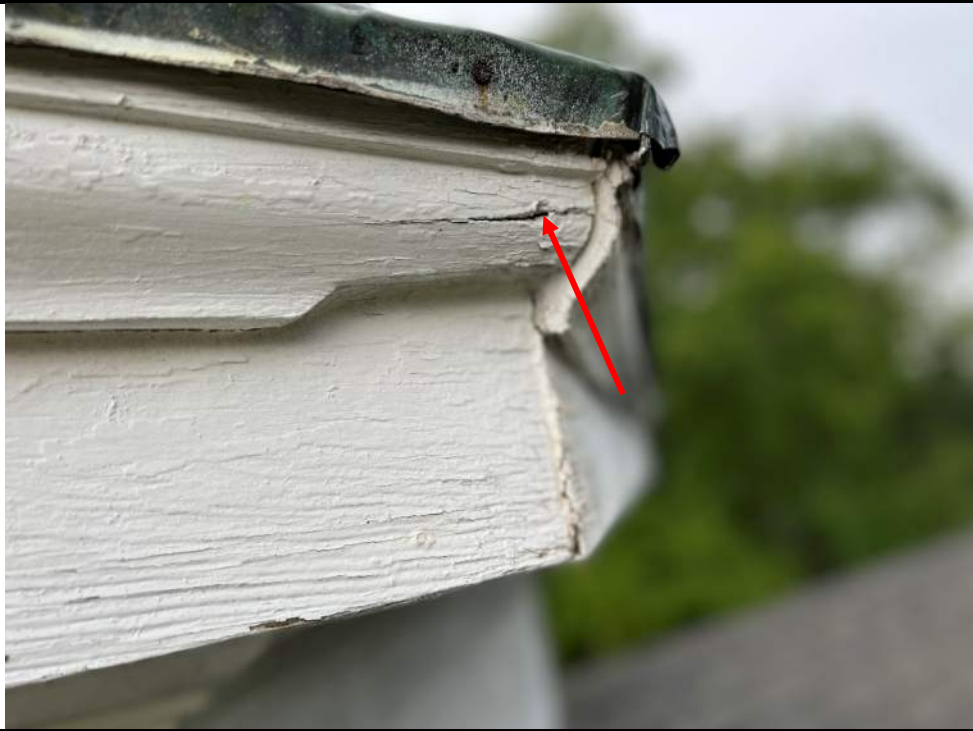
Photo 79: Wood trim at eaves and fascia exhibit paint peeling and some cracking
