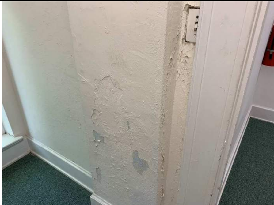
Photo 24: More observed peeling paint in wall near second floor fire escape doorway.
