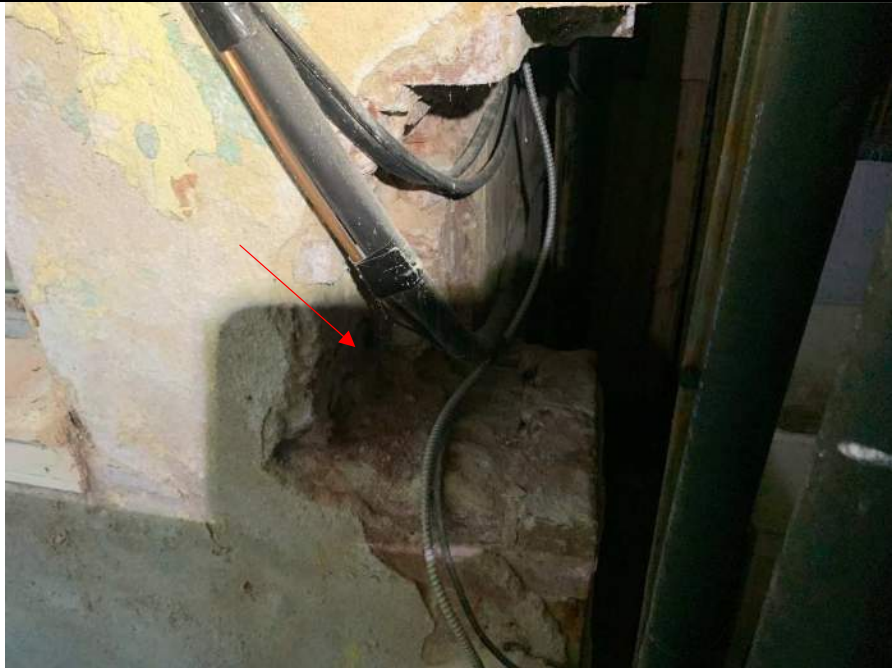
Photo 20: Existing wall/column section of ground floor mechanical room. Recommend fill in opening with similar brick material.
