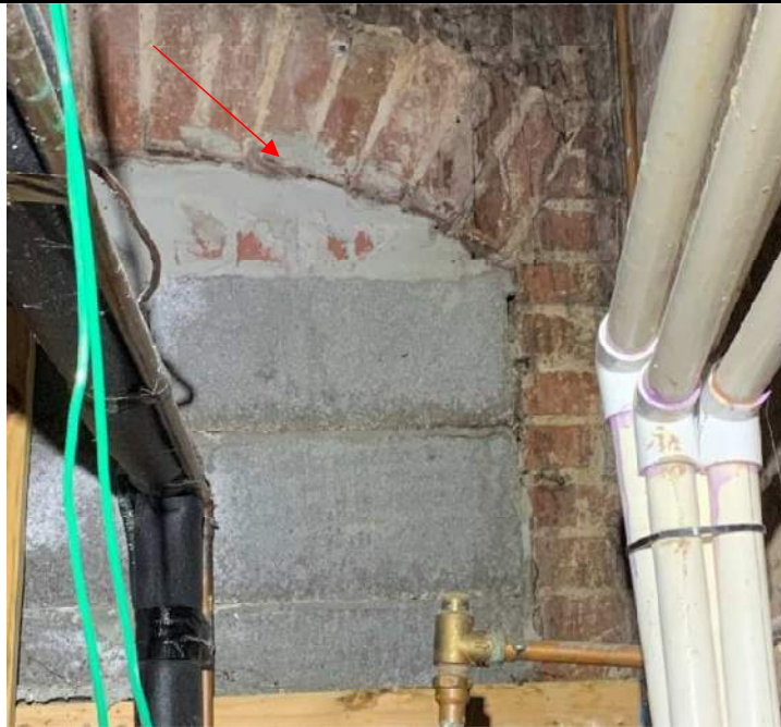
Photo 21: Observed crack/separation in previously filled in ground floor window.
