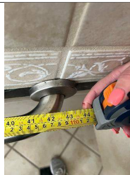
PHOTO #48: 42" Grab bar located in men's restroom on second floor (Compliant).
