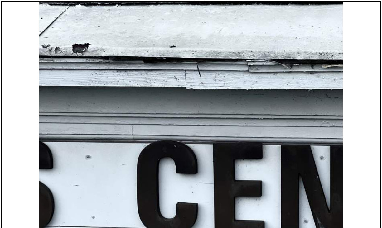
Photo 83: Exposed edge of wood substrate.
