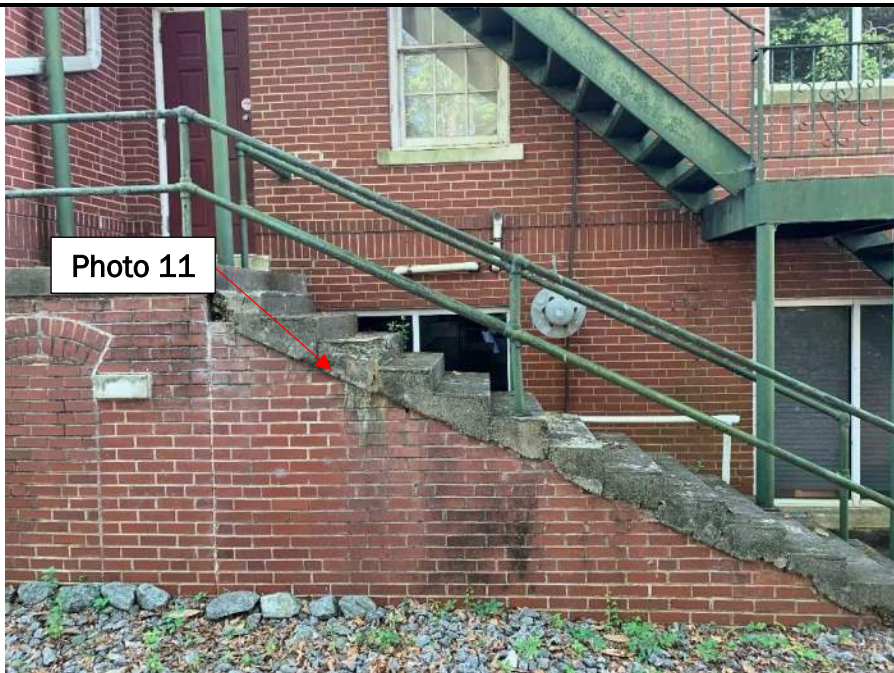
Photo 10: Side View of previous stair. Note brick and concrete spall distress.
