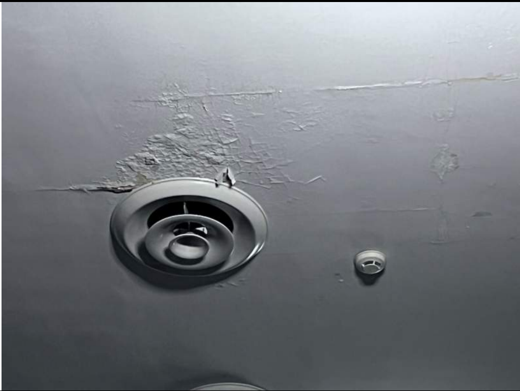
Photo 4: Blistered and peeling paint at suspected leak locations
