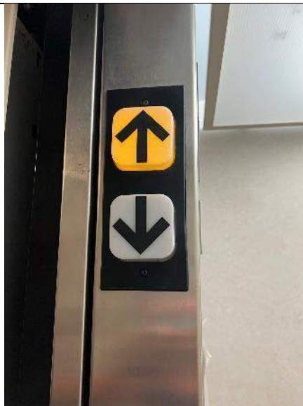
PHOTO #27: Audible and visual floor indicators. (Compliant).
