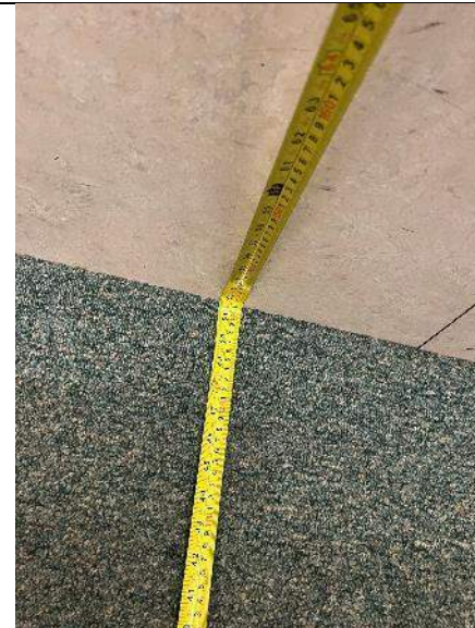
PHOTO #32: Elevator cab measurements 69" x 51" (Compliant).
