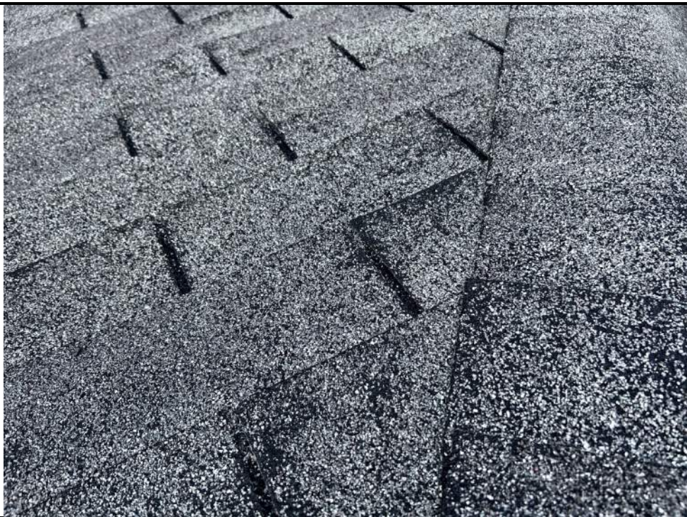
Photo 70: Erosion of ceramic granules from shingle surface
