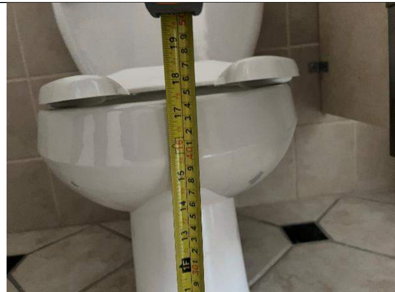
PHOTO #40: Toilet height of 18" in women's restroom second floor (Compliant).
