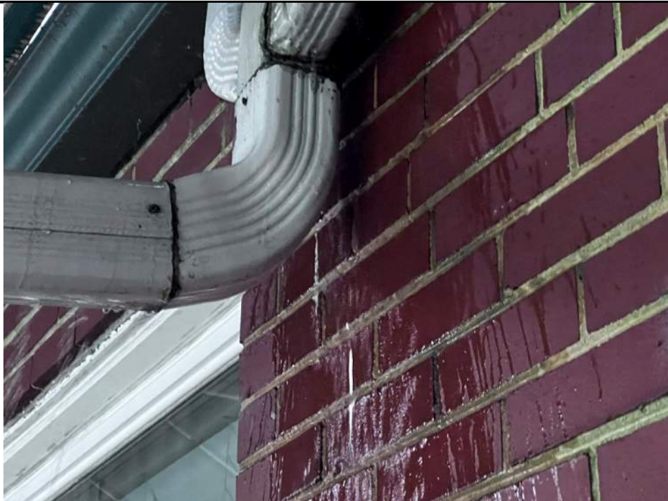
Photo 81: Capacity of main downspout insufficient with the additional gutter tie-ins.
