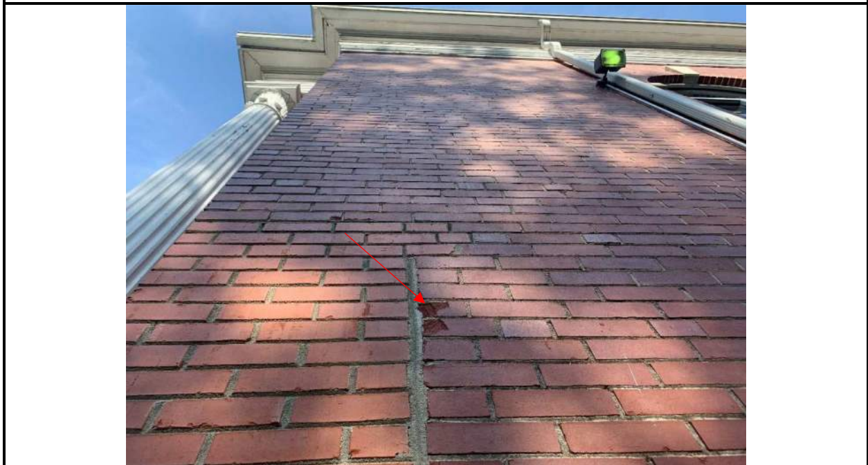
Photo 6: Typical exterior brick spall damage. Recommend replace damaged brick.
