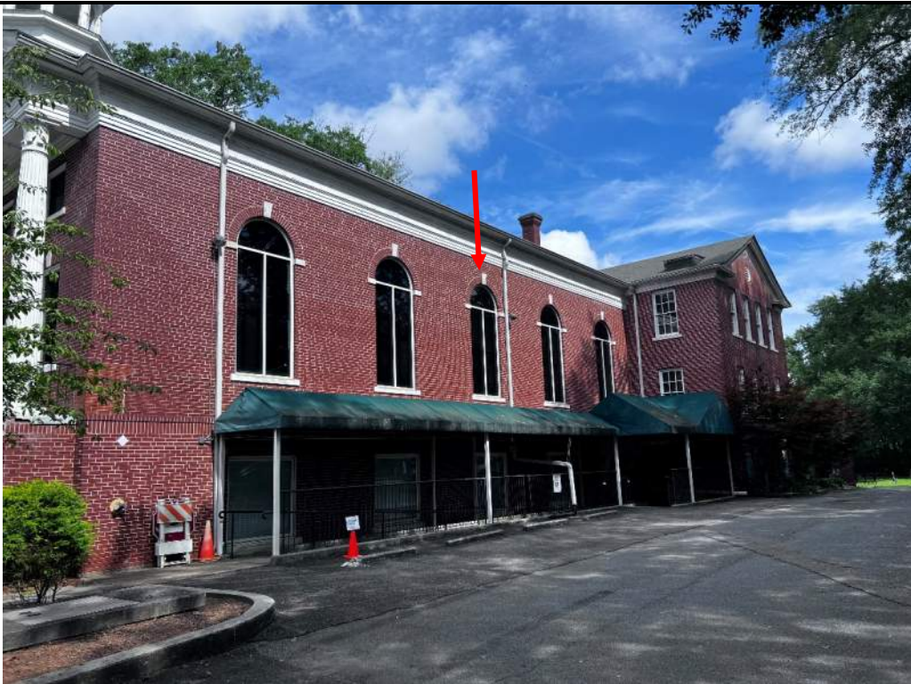
Photo 28: Overview east elevation, arrow points out keystone believed to be loose
