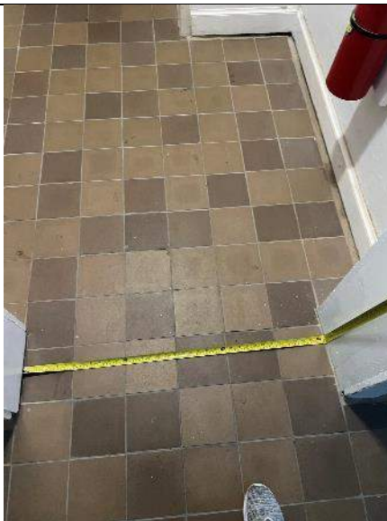
PHOTO #59: 36" opening on accessible route in building (Compliant).
