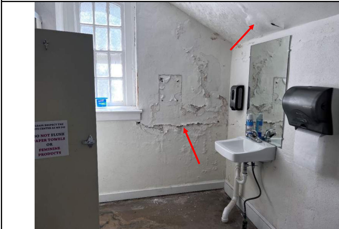
Photo 6: Blistered paint filled with efflorescence, south women's restroom, located below from exterior stairs
