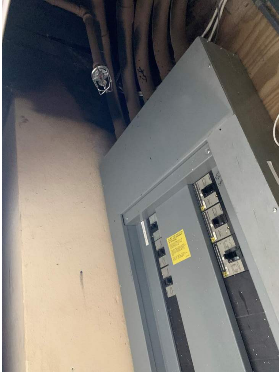
Photo 12: Sprinkler Head Over Electrical
