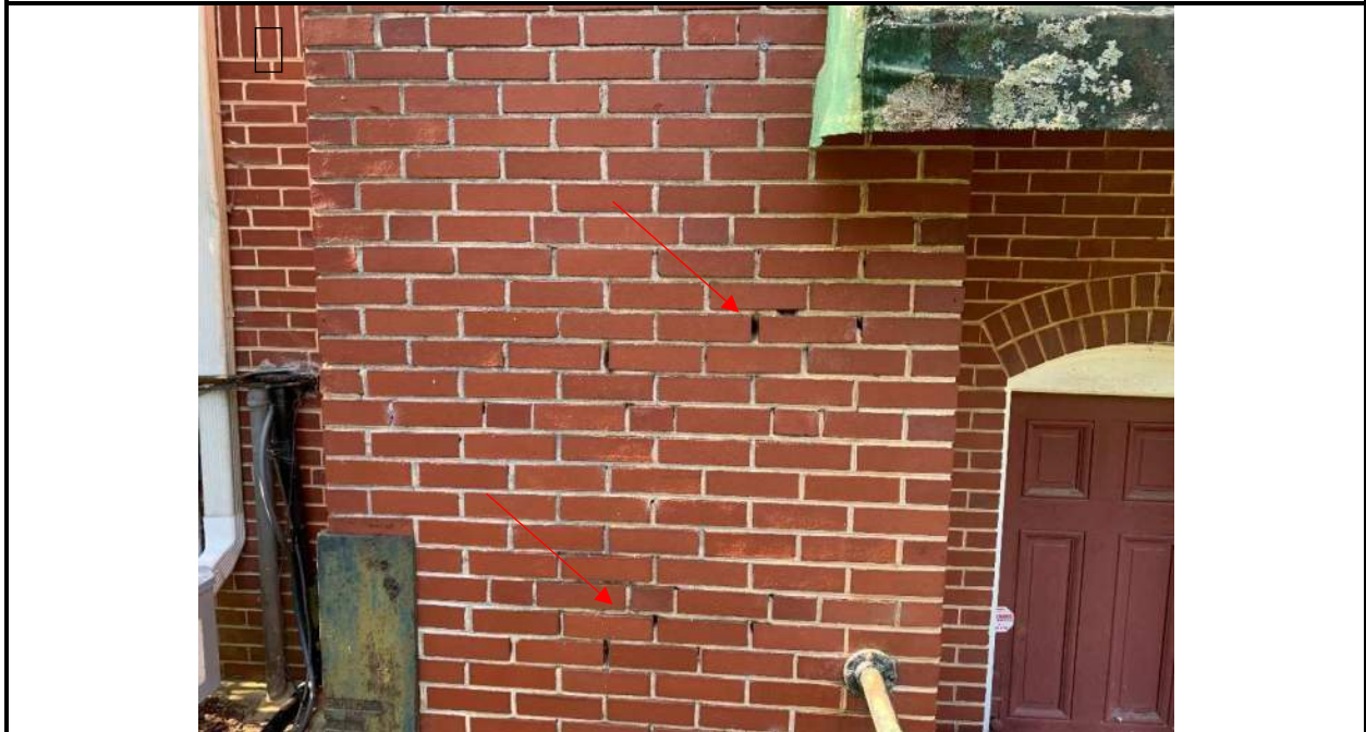
Photo 7: Typical mortar loss between exterior masonry brick. Tuckpoint repair recommended.
