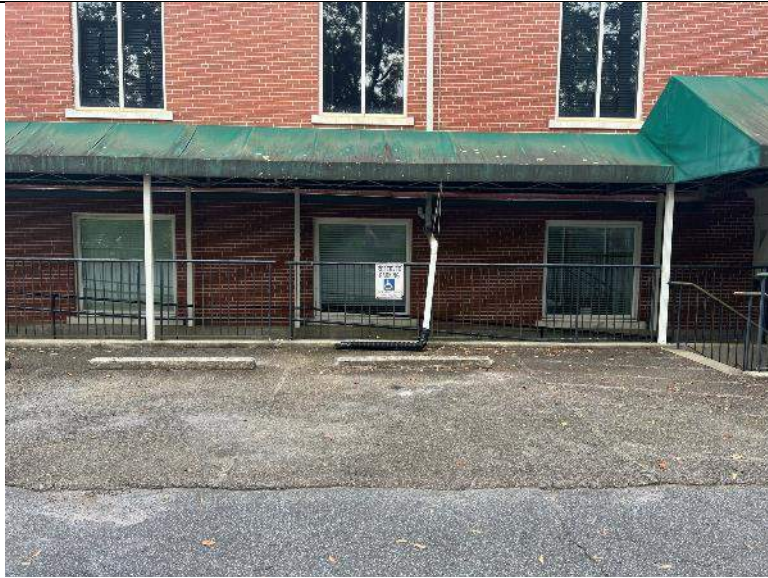
PHOTO #13: Designated accessible parking space. Note, it is not provided along the shortest accessible route and requires user to walk behind other vehicle to get to accessible route. (Non-Compliant).
