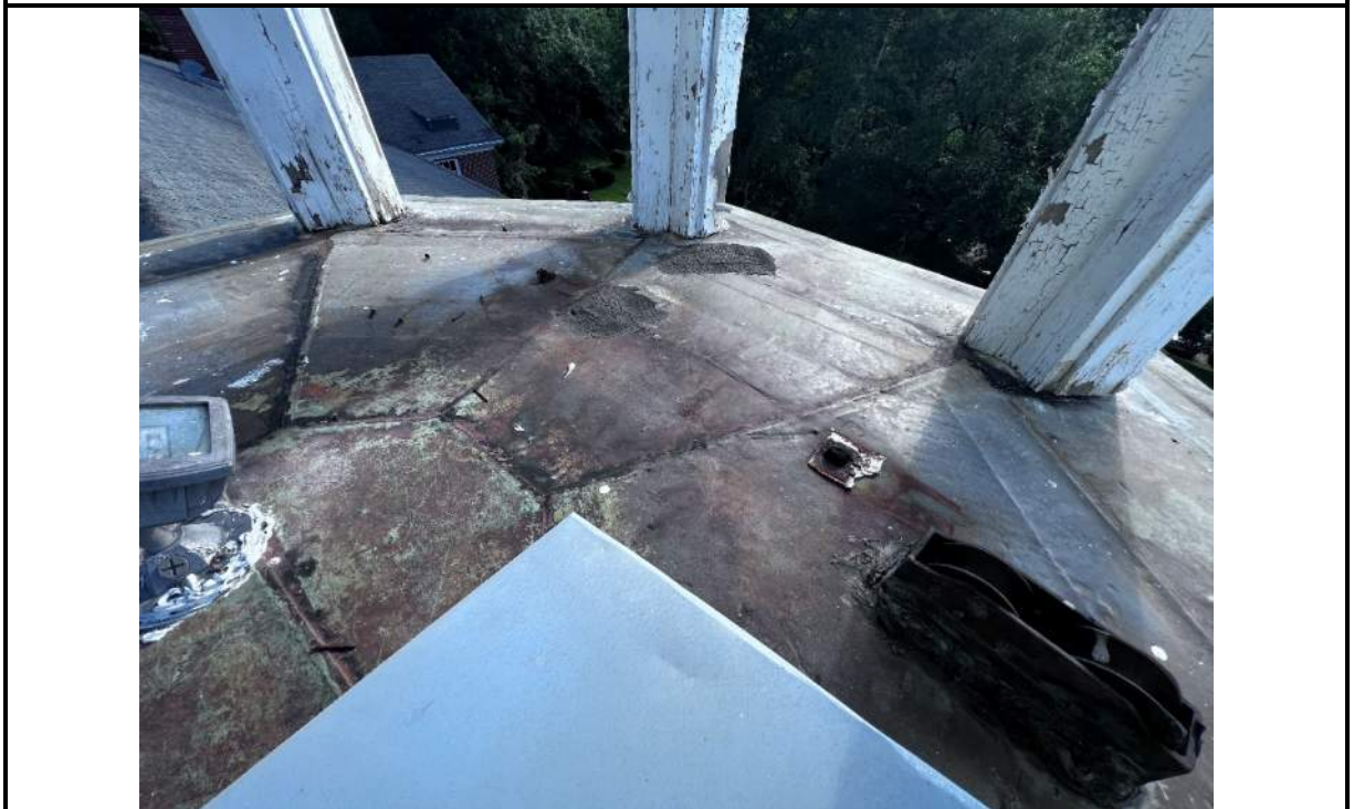
Photo 56: Overview of steeple exterior floor, bell pulleys still in place
