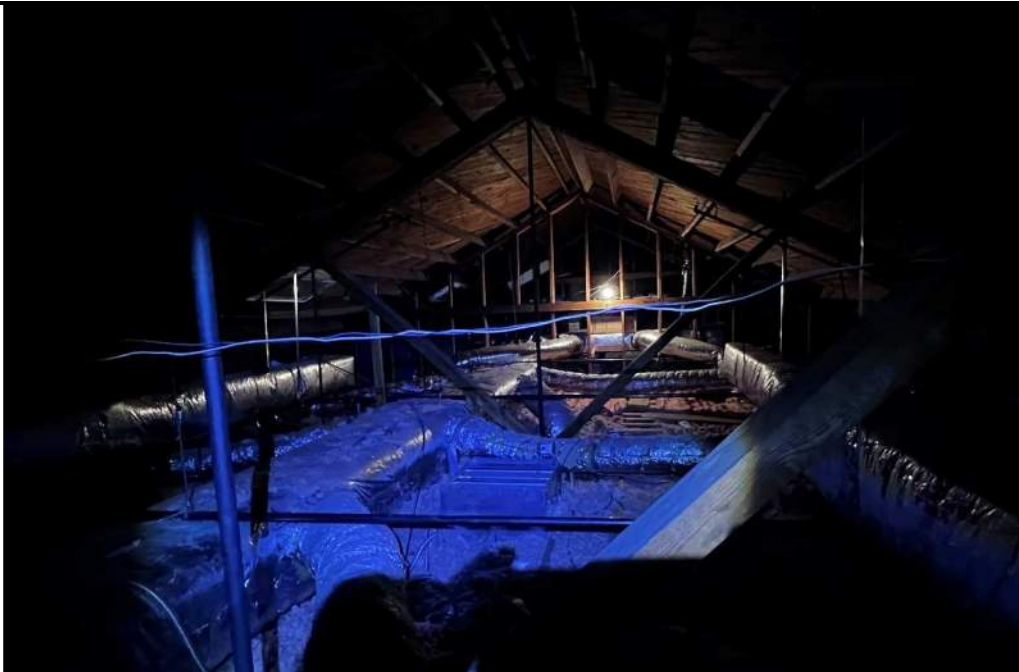
Photo 29: Overview of the underside of the roof deck framing, timber trusses, and wood joist. Note, truss components appear to be in good structural condition with observed signs of previous water infiltration near the steeple framing.
