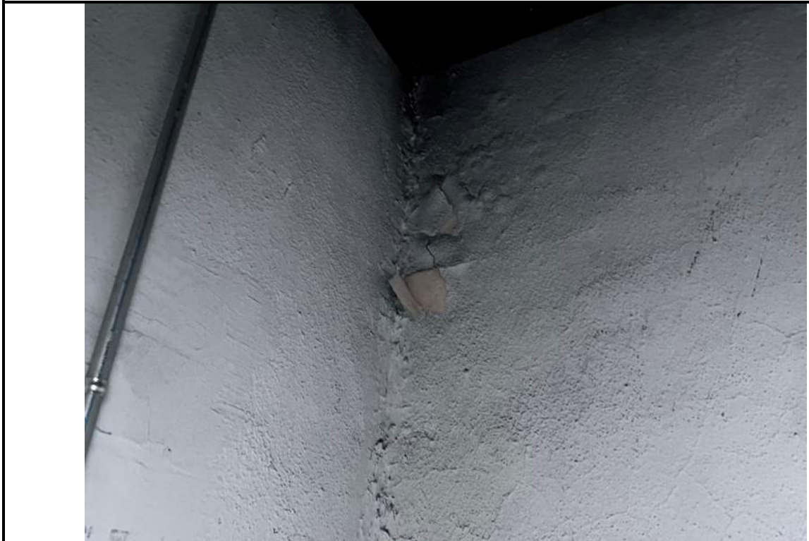
Photo 18: Blistered and peeling paint
