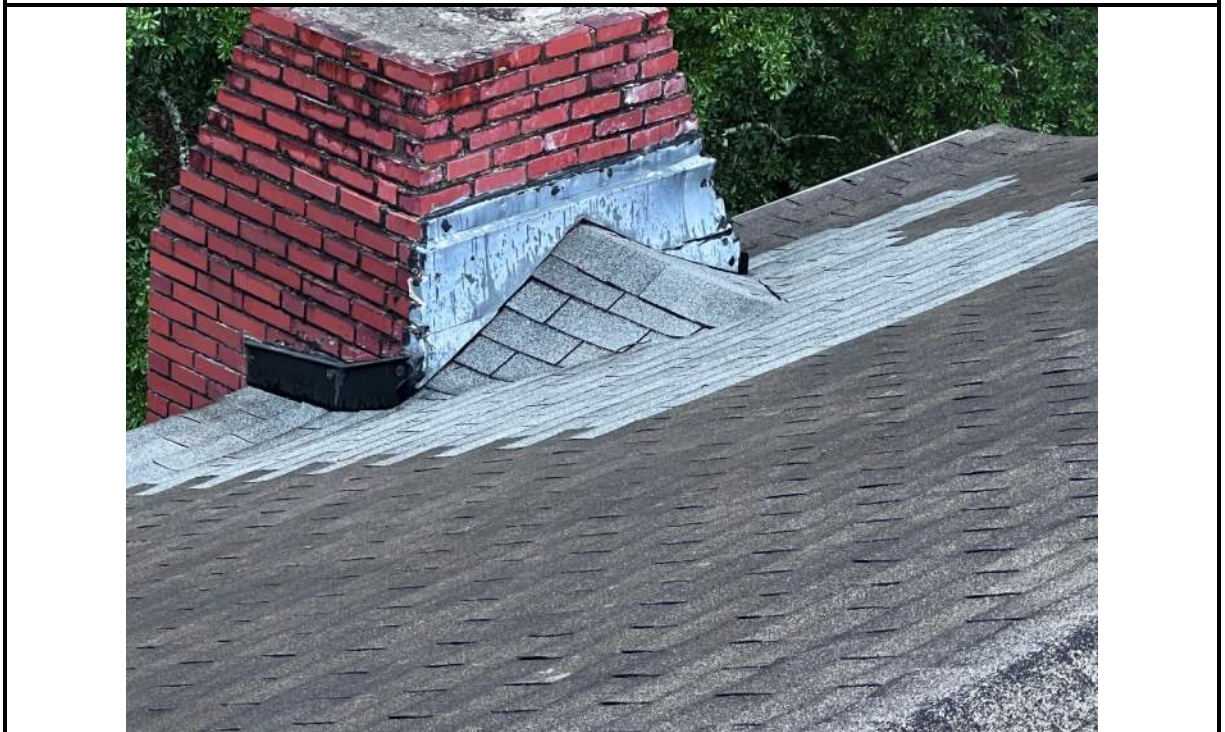
Photo 76: Location of previous roof repairs
