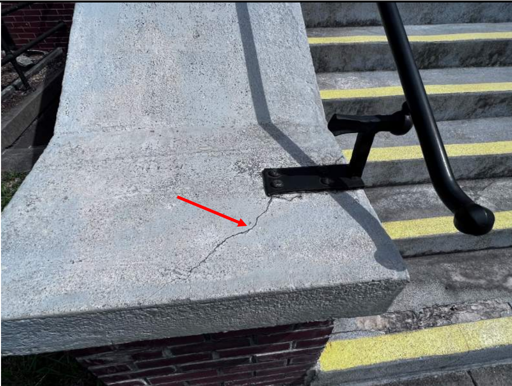
Photo 20: Cast concrete coping crack
