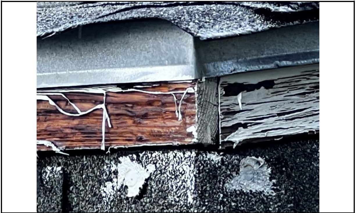
Photo 75: Exposed and deteriorated wood on 3-sides of popped up area
