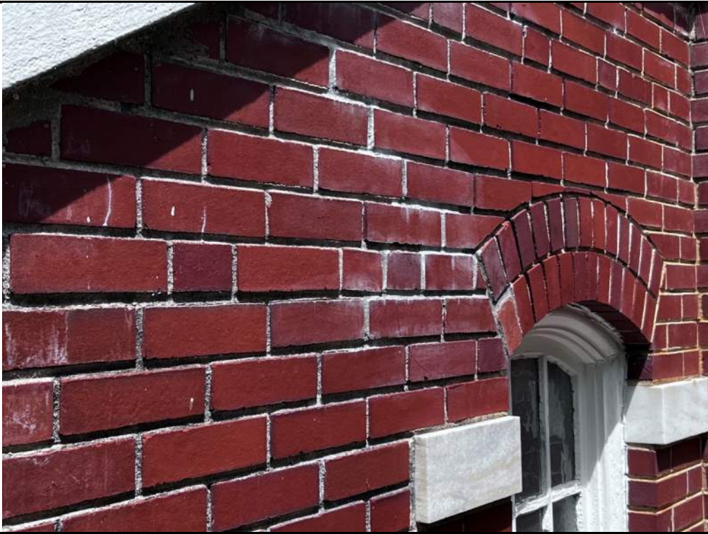
Photo 23: Appears to be previous mortar repair
