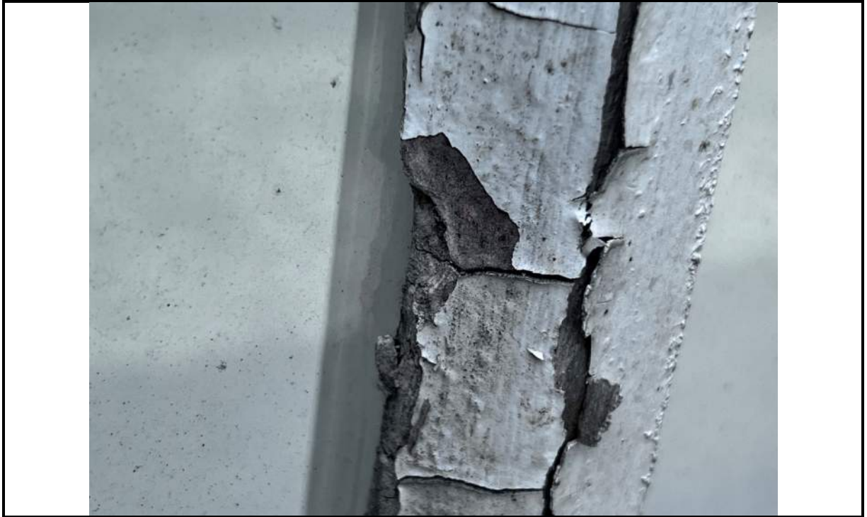
Photo 49: Glazing putty deterioration, typical condition most wood framed windows
