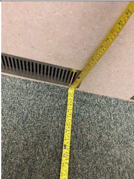
PHOTO #31: Elevator cab measurements 69" x 51" (Compliant).
