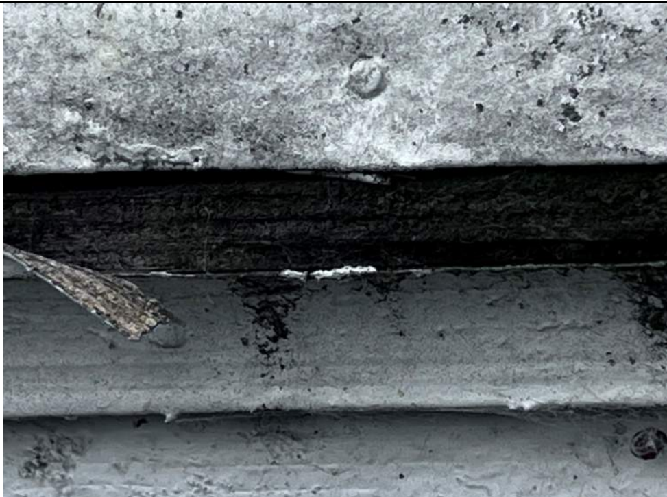
Photo 86: Exposed wood at edge of cornice metal.
