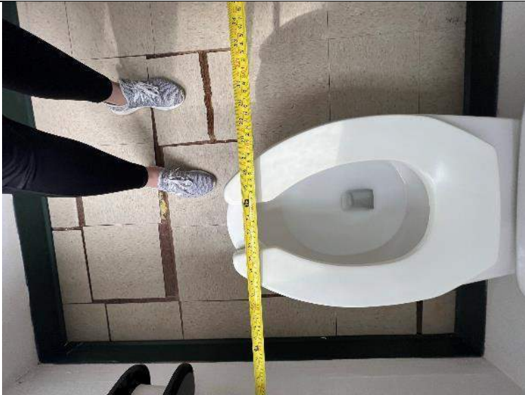
PHOTO #57: Toilet center is 22" from wall (Non-Compliant). Should be between 16-18".
