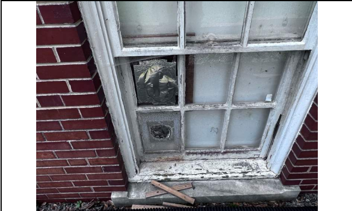
Photo 45: Vision lite openings infilled with metal, penetrations abandoned and taped over
