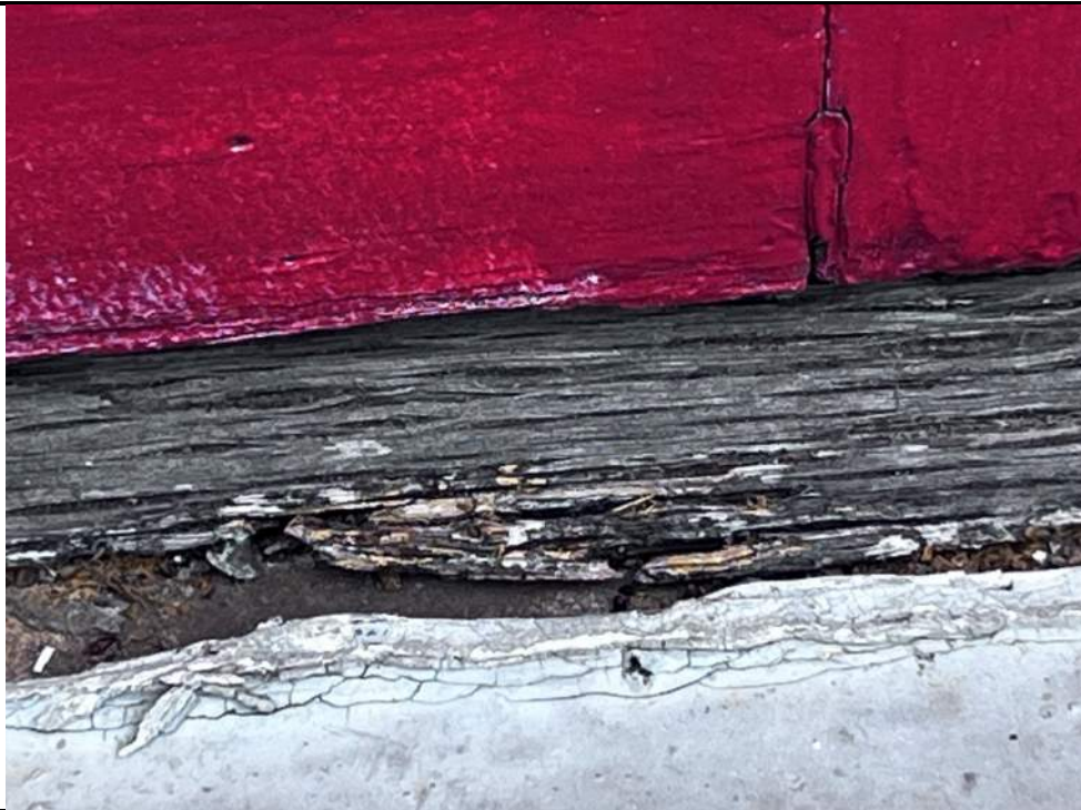
Photo 53: Threshold sill below door exposed and rotted
