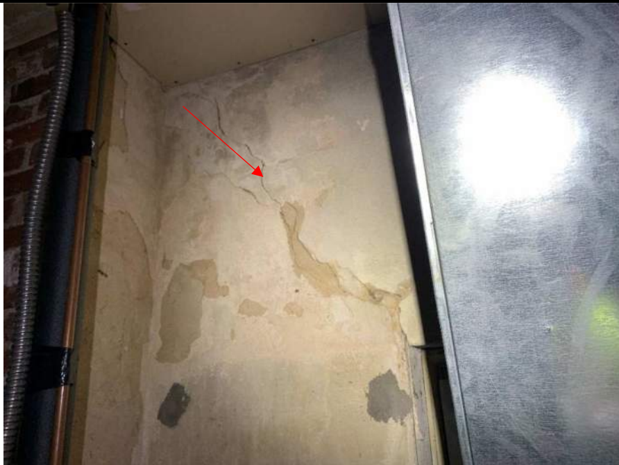
Photo 22: Typical cracks/separations and peeling paint in perimeter walls.
