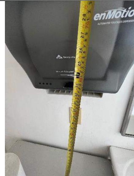
PHOTO #58: Paper-towel holder mounted too high for over an obstruction.
