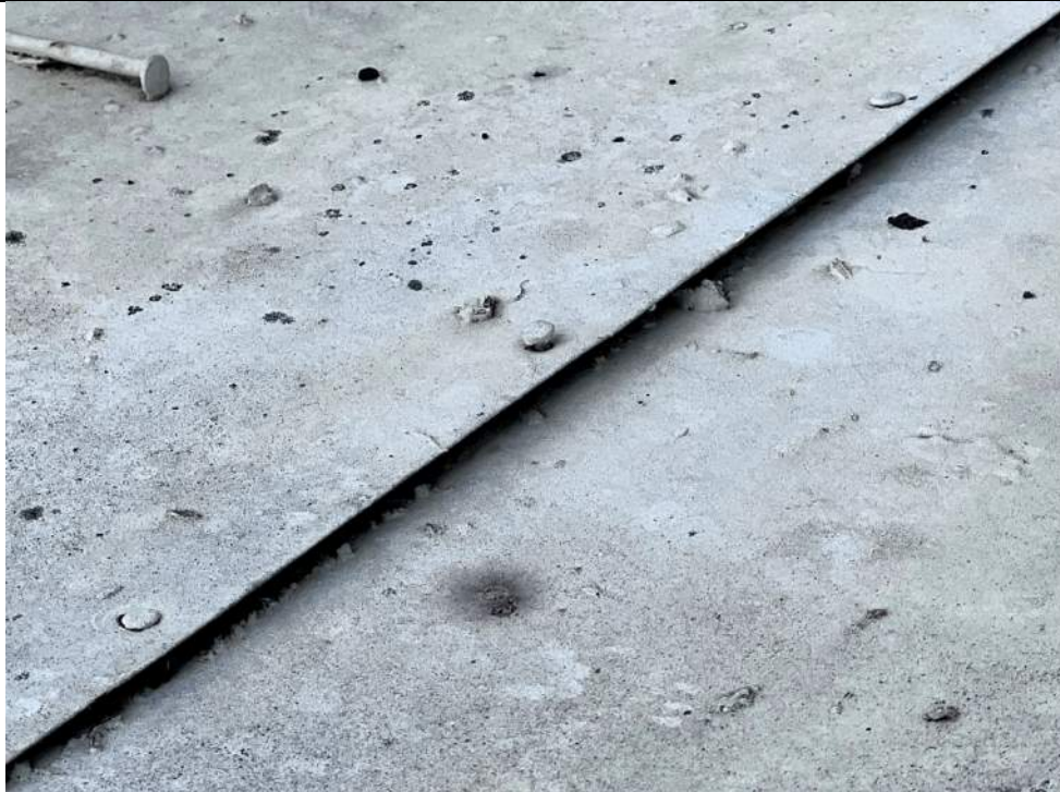
Photo 85: Open metal lap on cornice metal.
