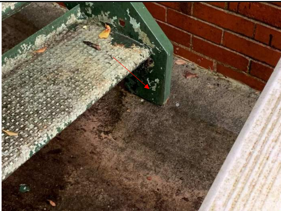
Photo 14: Previous steel fire escape connection to concrete slab on grade. Note, peeling paint. Recommended clean, prime, and paint steel staircase.
