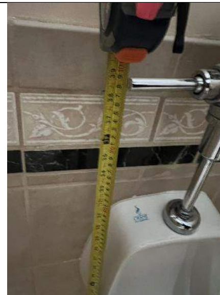
PHOTO #46: Urinal handle at 39" in men's restroom on second floor (Compliant).
