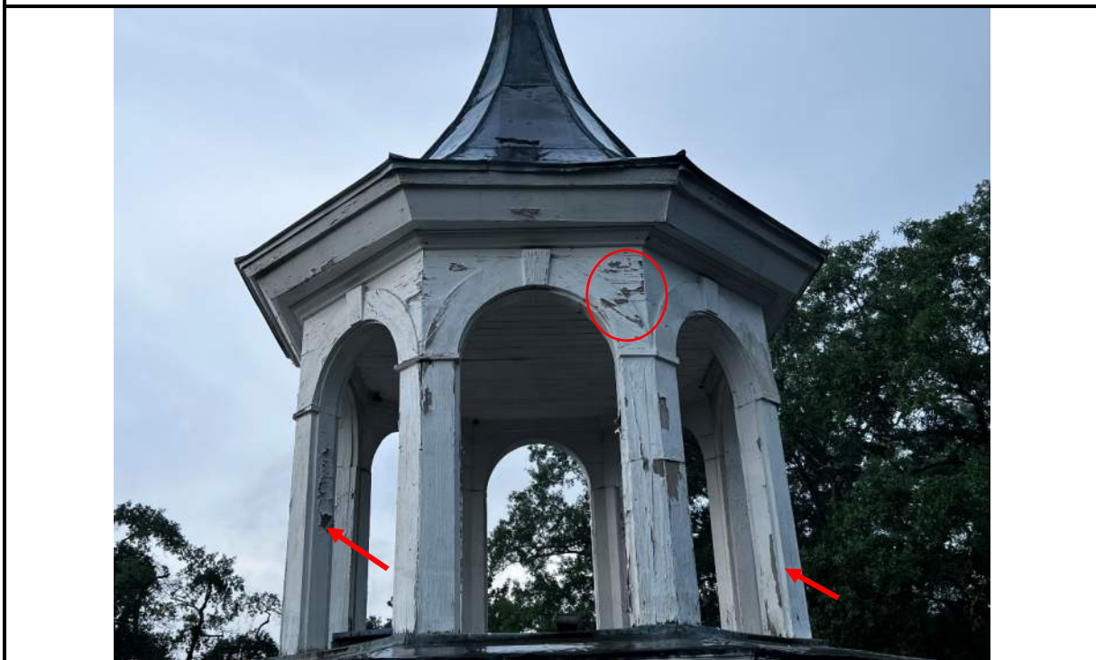
Photo 60: Overview of conditions typical all sides, paint in poor condition and exposed wood causing checking and cracking of the wood.
