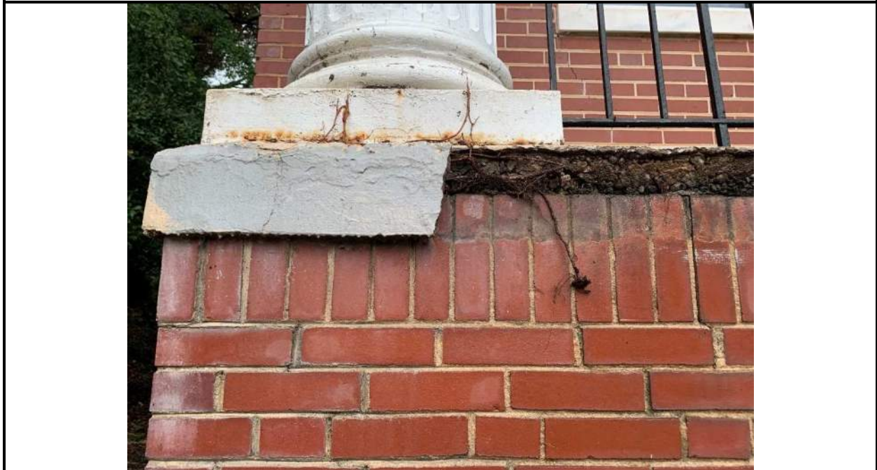
Photo 5: More Observed missing elevated concrete slab material and brick facade near south main entrance columns.
