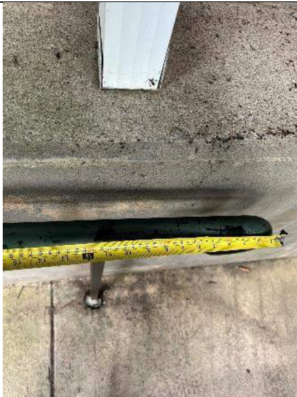
PHOTO #11: Railings include 12" overhang (Compliant).
