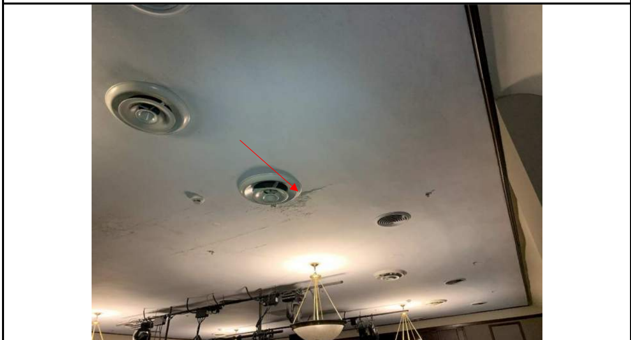
Photo 26: More observed second floor peeling paint in ceiling of theatre room. Possible water infiltration related damage.
