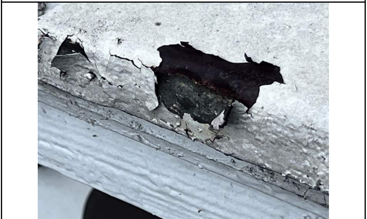
Photo 84: Isolated areas of metal corrosion on cornice return.
