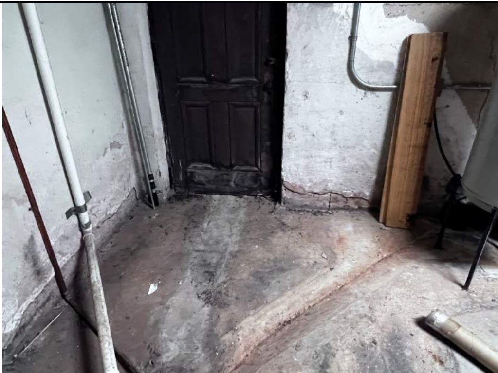
Photo 2: Interior view of mechanical room, note cracked plaster and efflorescence.
