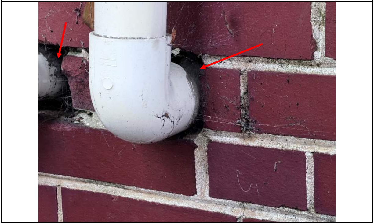
Photo 39: Unsealed pipe penetrations
