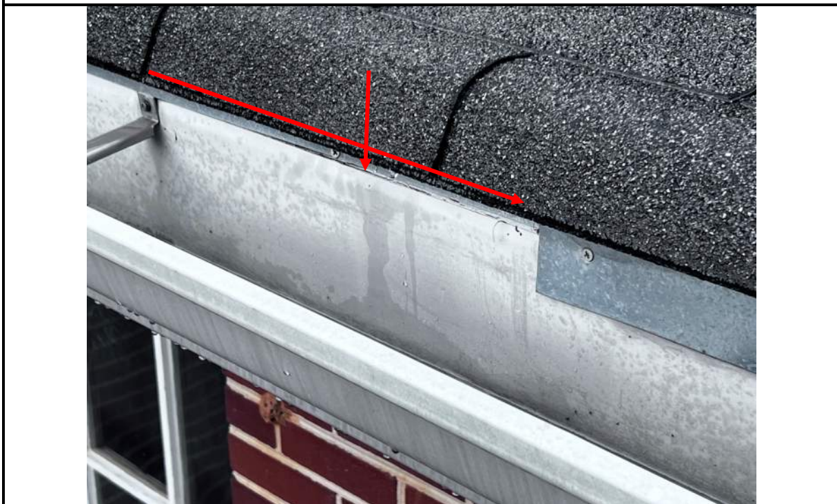
Photo 64: Shingle or edge metal does not cover the exposed top edge of gutter, roof may drip at this location
