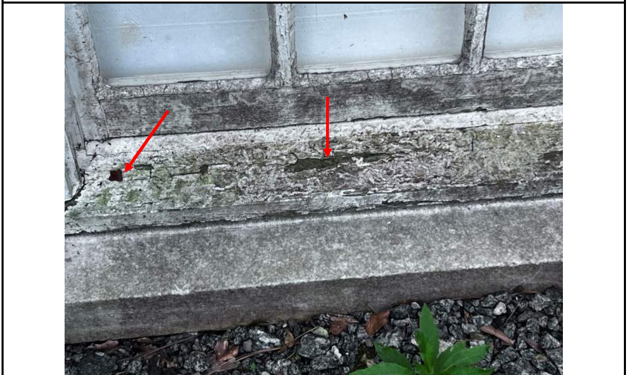
Photo 48: Deteriorated wood sill below window
