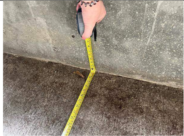
PHOTO #10: Ramp width is 60". (Compliant).
