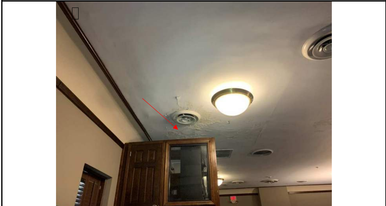
Photo 25: Observed second floor peeling paint in ceiling of theatre room. Possible water infiltration related damage.
