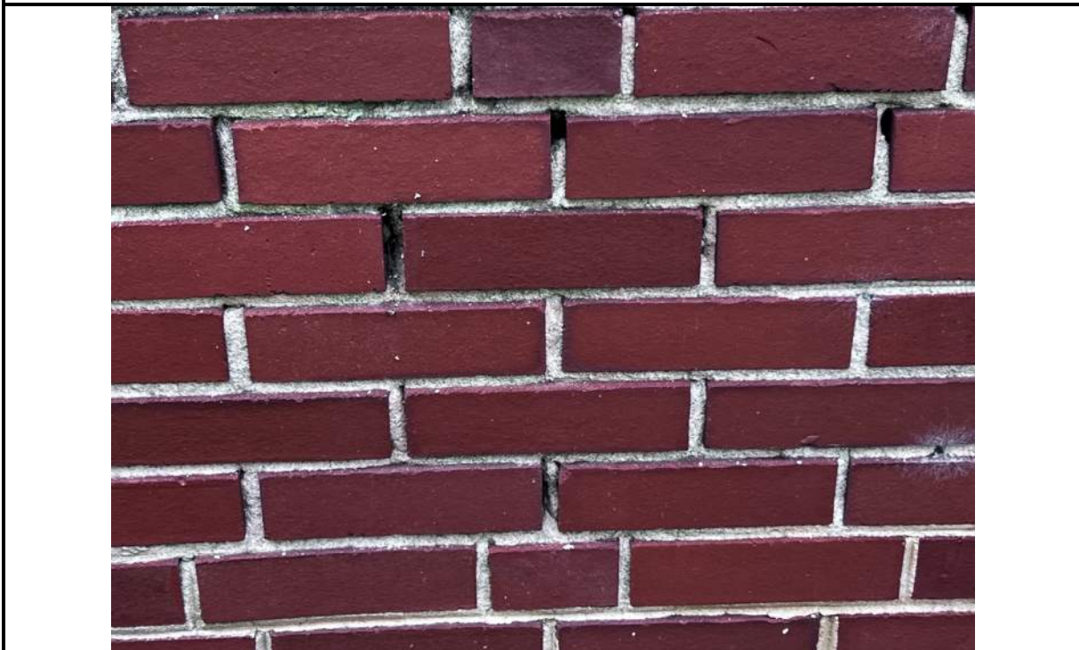
Photo 38: Eroded and missing mortar, in vicinity of wall damage in basement level mechanical room
