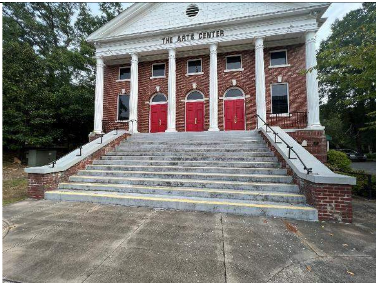
PHOTO #23: Alternate entrance – non accessible. Directional signage should be posted directing to accessible entrance.
