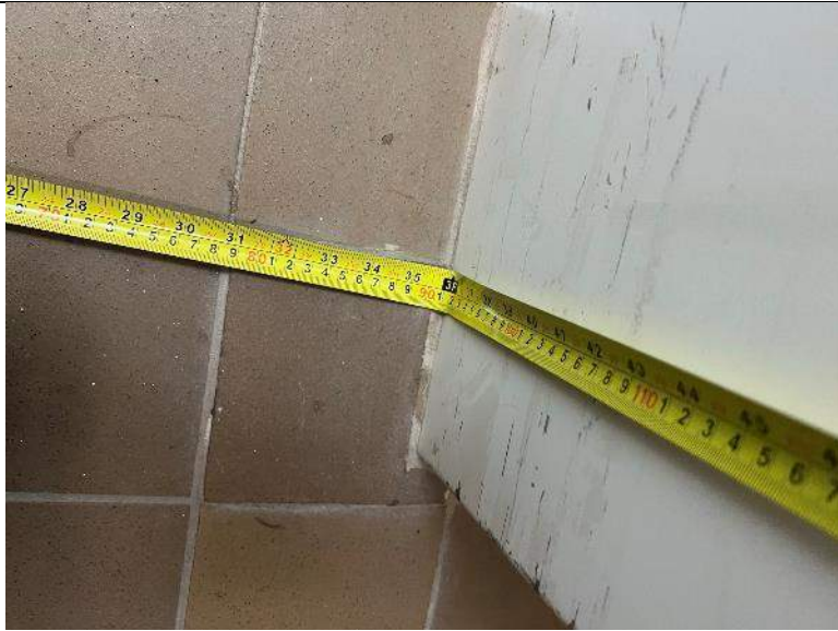
PHOTO #25: Elevator opening width is 36" (Compliant).
