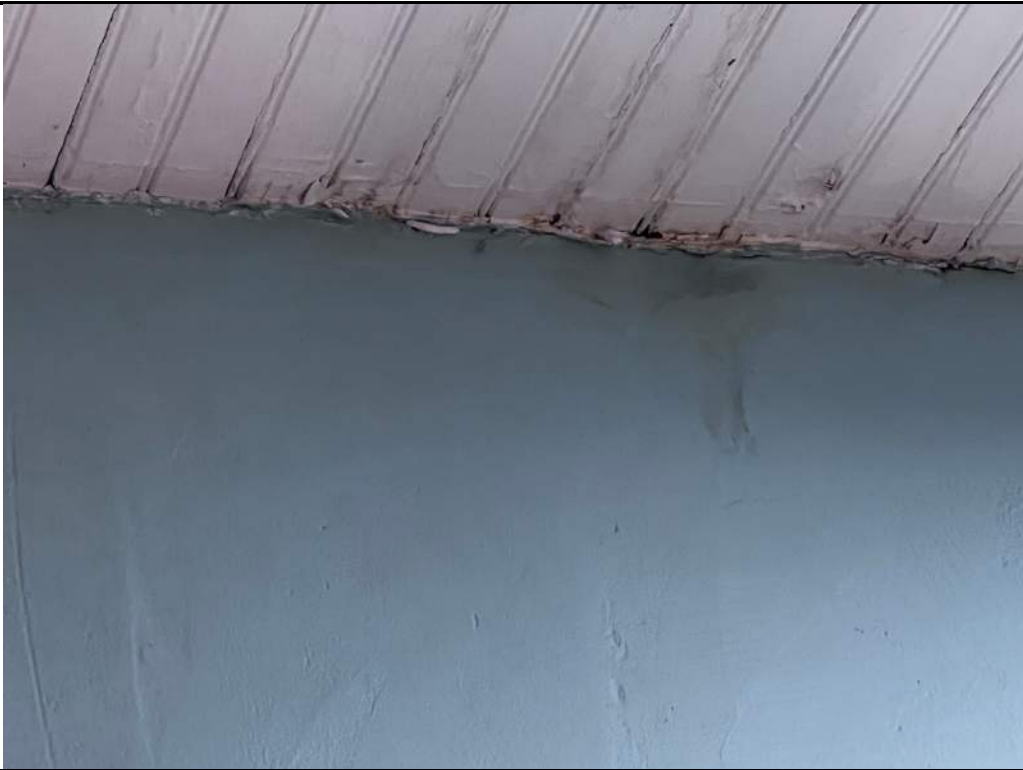
Photo 13: Beadboard ceiling exhibiting previous moisture damage
