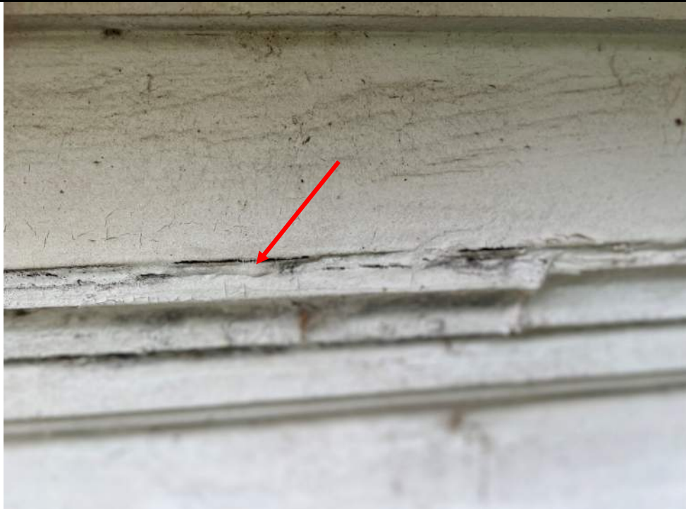
Photo 80: Wood trim at eaves and fascia exhibit paint peeling and some cracking
