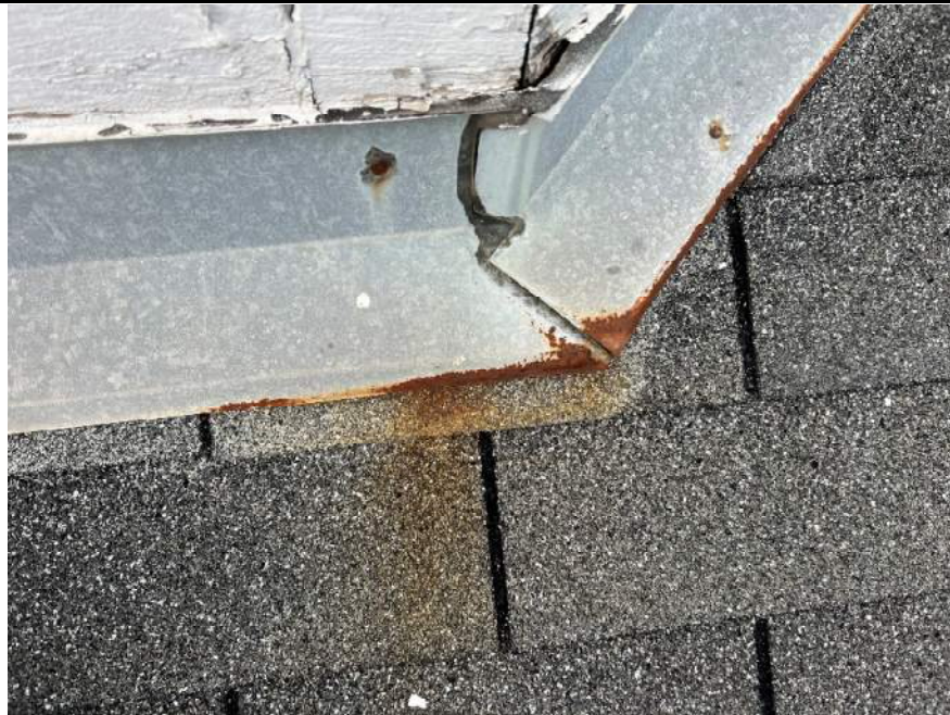
Photo 65: Metal cornice return cap exhibits some corrosion
