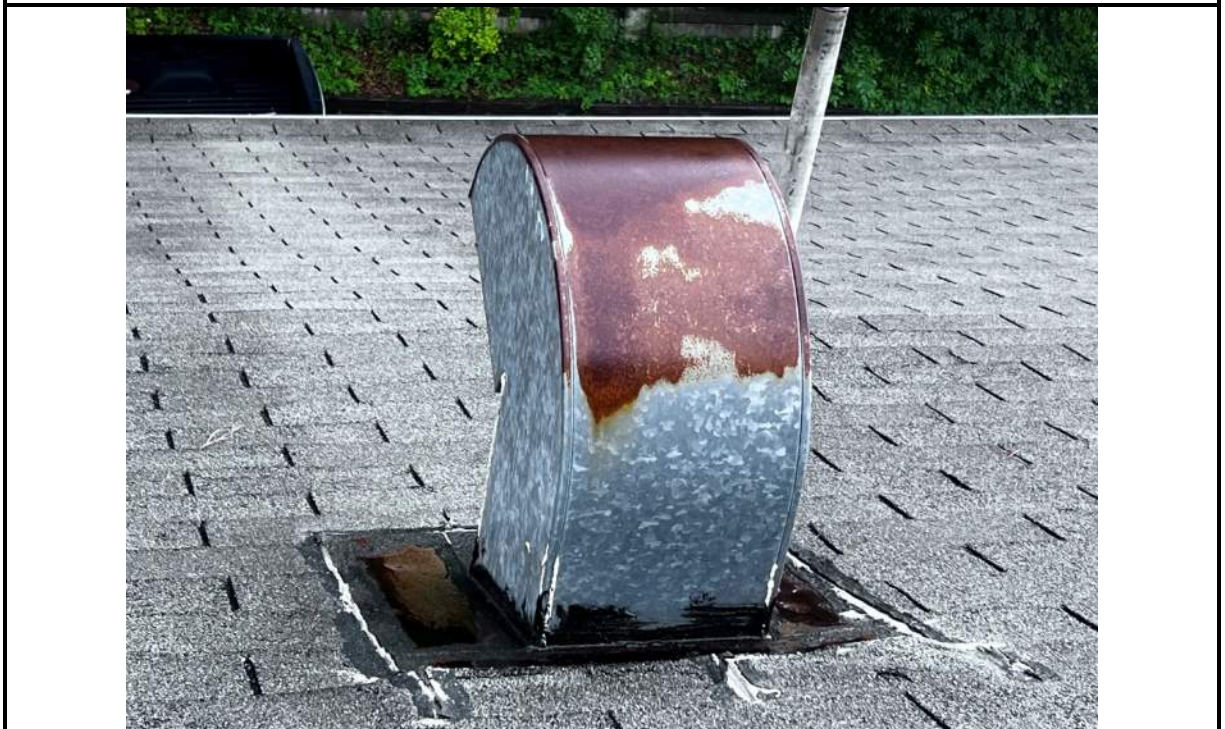
Photo 78: Metal component surface corrosion
