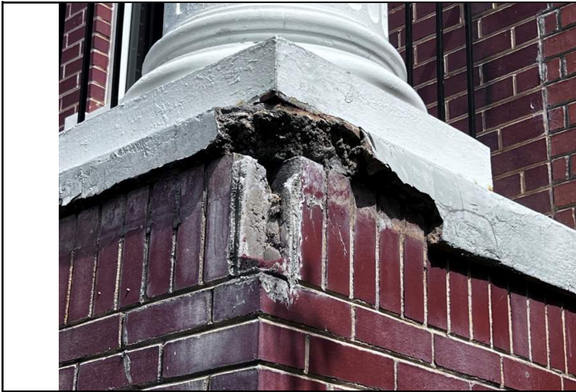
Photo 25: Concrete deck at entrance, above restrooms, is spalled.
